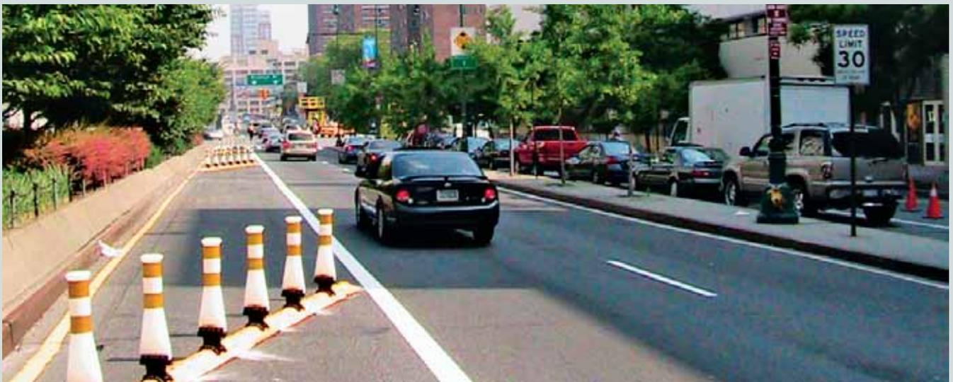
Flexible delineators installed in left lane on northbound Adams Street to prevent left turns onto westbound Tillary Street.
