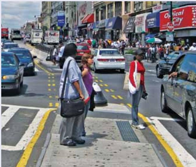
Construction of two new pedestrian refuge islands on E. 149<sup>th</sup> Street, reduced a 60 foot crosswalk into two 25 foot sections.
