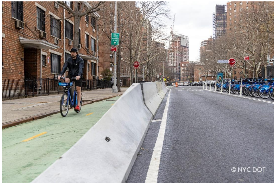
Bike lane hardening at Clinton Street, Manhattan
