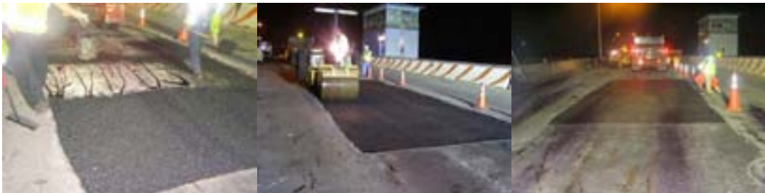
Belt Parkway Bridge over Mill Basin: Installation of New Asphalt. Compacting the Asphalt With the Assistance of a Gasoline Roller Engine From the Roadway Repair and Maintenance Division. Completed Resurfacing Work. (Installation Credit: Yousef Demis, GRE Credit: Ali Mozaffari)
