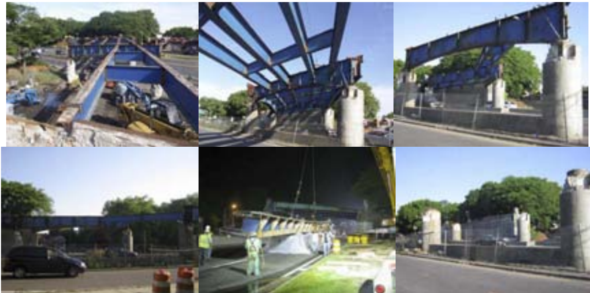
East 8 th Street Bridge Superstructure Steel Removal in June 2010. Loading a Fascia Girder on a Trailer. North View After Completion of Steel Removal.
