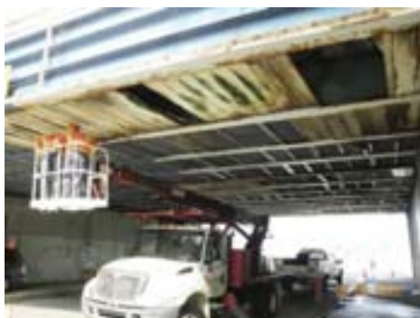
2009 Inspection: The Entire Underside of the Bay Ridge Avenue Bridge Deck is Shielded With Timber Planking and Steel Wire Mesh Netting. The Shielding was Temporary Removed to Perform the Inspection of the Deck. Shielding was Replaced After the Inspection. (Credit: NYSDOT)
