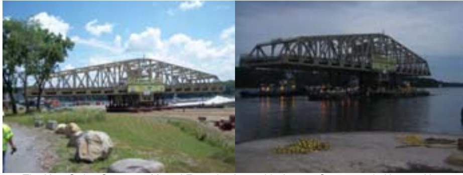
The New Swing Span was Moved From the Assembly Area at Coeymans in Upstate New York to the Twin Barges on July 11 and 12, 2010. It was Then Delivered by Barge to the Contractor Facility in Jersey City, New Jersey on July 14.
