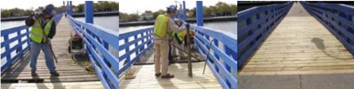
Replacing Planks on the Ocean Avenue Bridge: Carpenters John Green, Mark Pavia, Michael Short, and Andrew Myjer. (Credit: Pinakin Patel)
