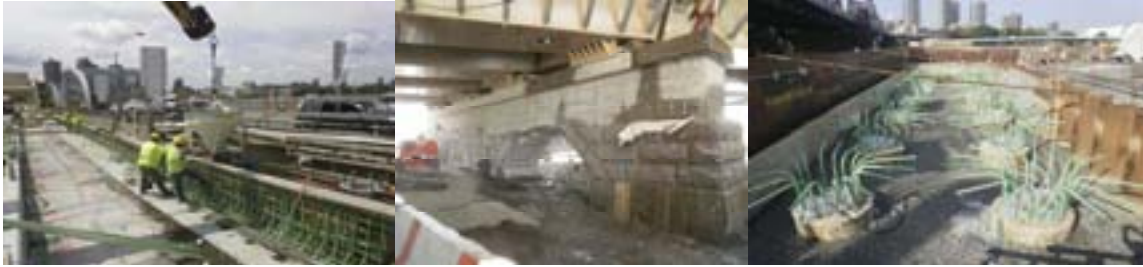
August 2010: Finished Placement of High Friction Concrete for Overhead Sign Structure at Span 9. Setting and Grouting Granite Stone Facing at Pier 8. Finished Placement of Caisson Concrete to New Higher Elevation at Bronx Relieving Platform "B".
