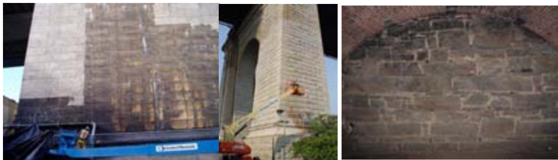
Cleaning the Masonry of the North Face of the Manhattan Bridge's Brooklyn Anchorage and of the North and East Faces of the Roosevelt Island Pier of the Queensboro Bridge. Masonry of the East Drive Bridge Over Eastwood Arch.
