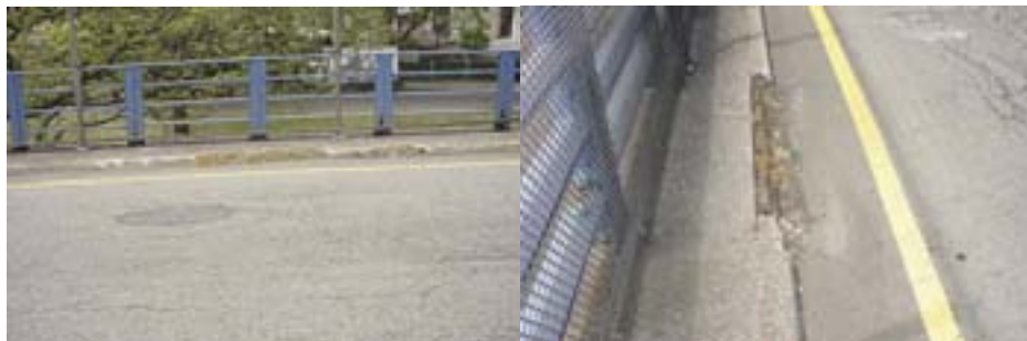
Spalled Section of Curb on the East 8 th Street Bridge in 2006. (Credit: NYSDOT)
