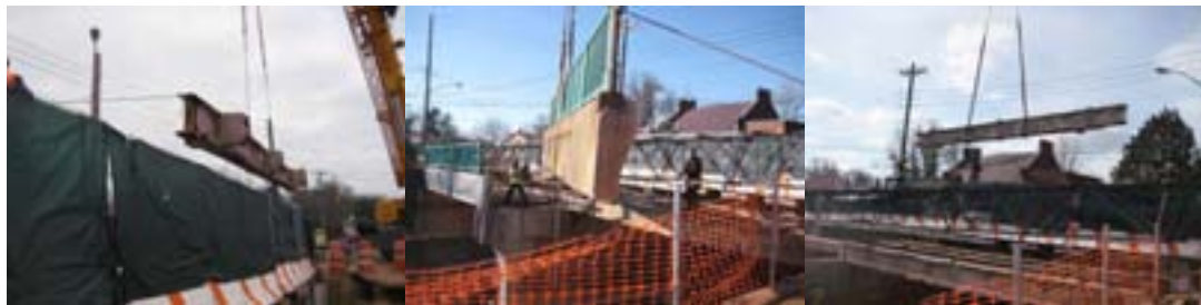
Annadale Road Bridge: Stage I Construction in February 2009. Placing a Temporary Truss to Support Utility Conduits. Removing the Eastern Bridge Railing Fence and the Stringer.
