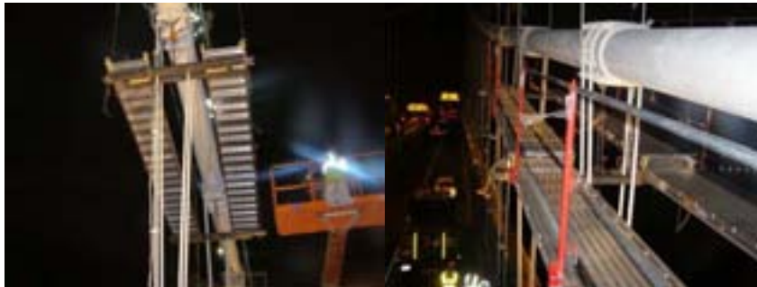
April 2010: Division Ironworkers Installed Scaffolding Along Cable "D" of the Brooklyn Side Span for the Field Test Phase of the FHWA-Sponsored Bridge Cable Corrosion Study. (Credit: Hany Soliman)
