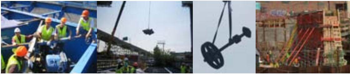
June 2010: Removing the Motor for Replacement and the Main Machinery Shaft for Rehabilitation. Oiler Carl Wharton, Mechanical Engineer Ibrahim Ibrahim, Oilers Tom Strommen and Richard Morreale, and Construction Project Manager Ali Mozaffari. (Credit: Vera Ovetskaya) September 2010: Steel repairs and concrete placement for the west abutment wall.
