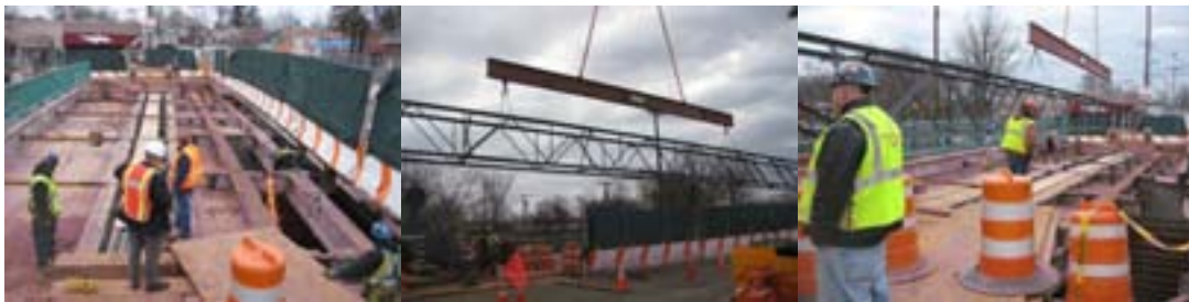
Annadale Road Bridge: Stage I Construction in February 2009. Saw Cutting the Diaphragms, Removing the Stringers, And Placing a Temporary Truss to Support Utility Conduits.
