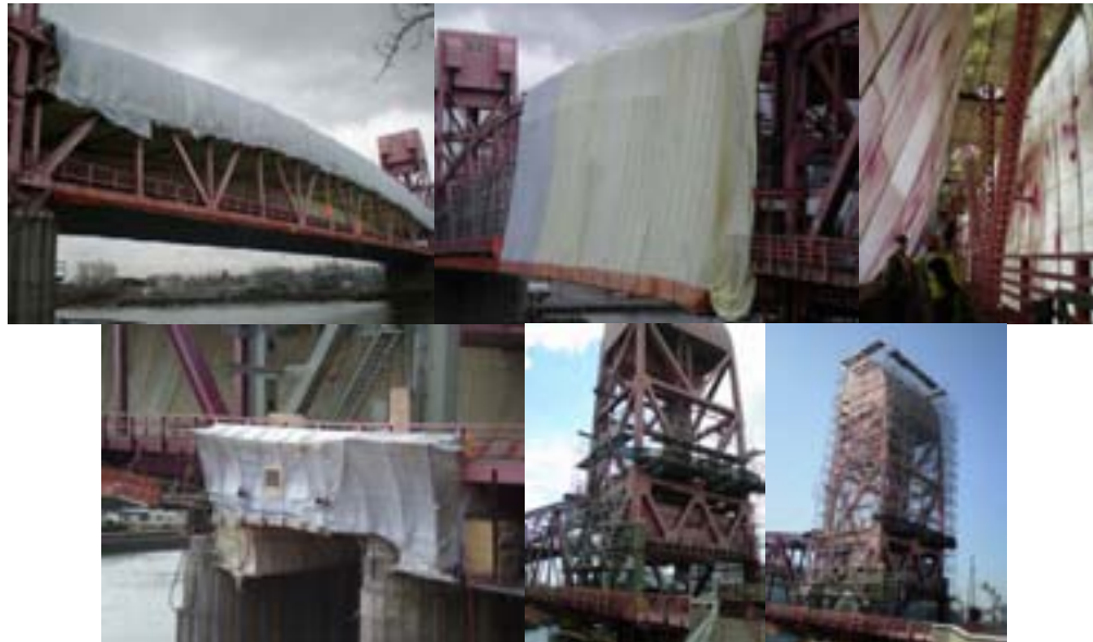
2008: Roosevelt Island Bridge Containment. Preparing the South Truss Containment. South Side of Main Span. Erecting Scaffold to Build Containment at the West Tower.
