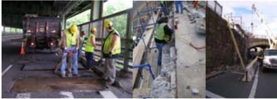
Replacing Asphalt Around a Plate on the 5 th Avenue Bridge in June 2010: Highway Repairer Robert Tuite, Bridge Repairer and Riveter Ignazio Trapani, and Assistant City Highway Repairers Umberto Fava and Thomas McKenzie II. (Credit: Joseph Flood) Cement Masons Repairing the Retaining Wall at the Southern Boulevard Bridge over East Fordham Road in November 2010. (Credit: Sohrab Hossain)
