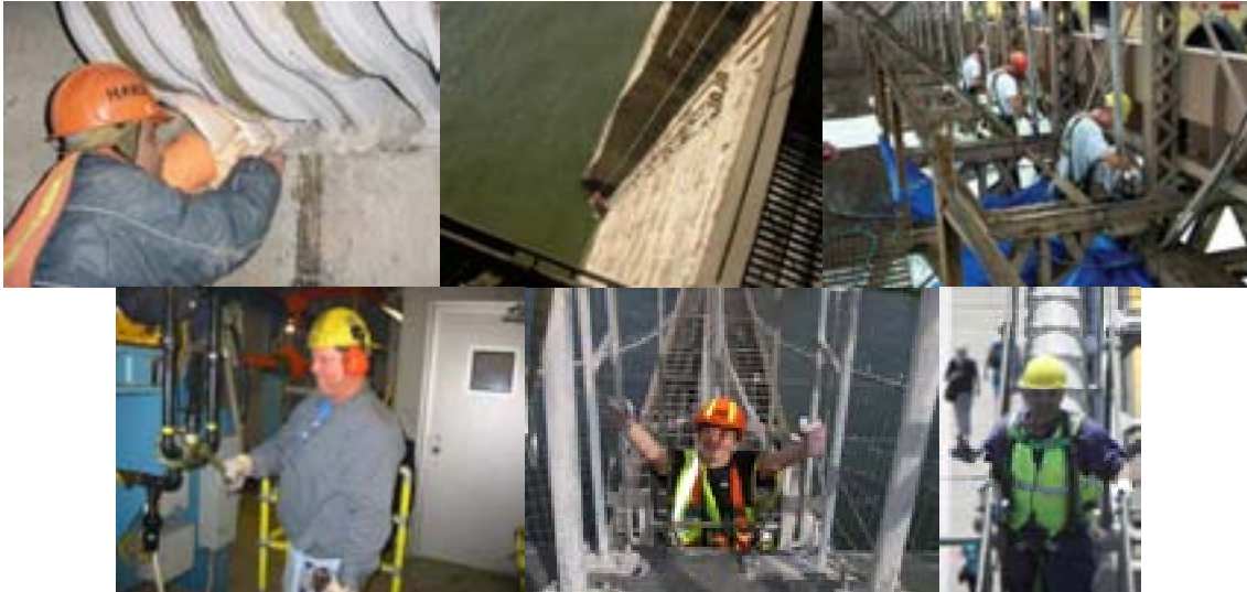
Inspecting the Eyebars in the Brooklyn Anchorage of the Manhattan Bridge. (Credit: NYSDOT) Repairing the Brooklyn Bridge Standpipe System, 130 Feet Below the Roadway. Maintenance Crew Conducting the Annual Cleaning and Lubrication of the Solid Rod Suspenders Spherical Bearings on the Brooklyn Bridge. (Credit: Anatoly Orlov) Oiler T. McAuliffe at the 9 th Street Bridge. Assistant Mechanical Engineer Vera Ovetskaya Climbing to the Brooklyn Bridge Tower in 2008. (Credit: Gennadiy Kaplun) Oiler Samuel Garcia Jr. Climbing the Brooklyn Bridge Cable in June 2010. (Credit: Thomas Whitehouse)
