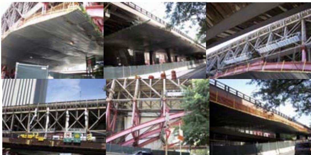
July 2010: Installation of the Platform for the Abrasive Blasting Operation at Franklin Square and the Containment Rigging at Pearl Street.
