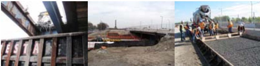
Rockaway Parkway Bridge in November 2010: Stage II Demolition of the Existing Bridge Concrete Deck. Overview of the Stage II Demolition. The Asbestos Abatement Operation is in the Foreground. The Installation of New PCC Roadway for the Westbound Off Ramp.
