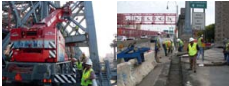
July 2010: Looking East at Damaged Brooklyn Tower (South Outer Roadway) Strut Replacement. October 2010: Looking East at the Lane 8 Precast Barrier Concrete Foundation Placement at Manhattan Plaza.
