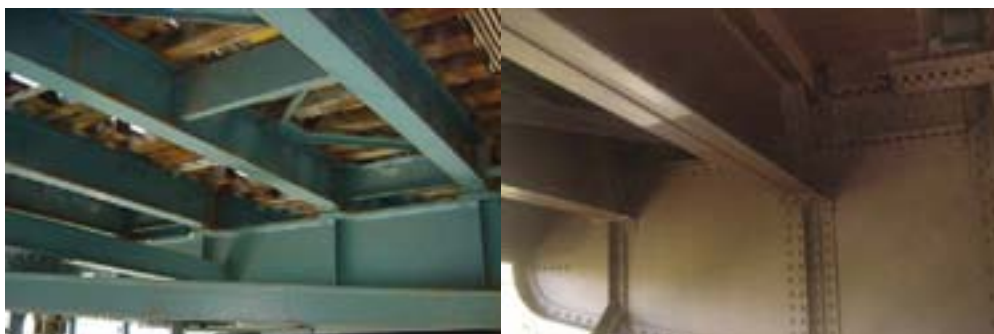
South Transit Floorbeams, Stringers, and Bracing Members on the Manhattan Bridge. Queensboro Bridge North Outer Roadway Floorbeam. (Credit: NYSDOT)
