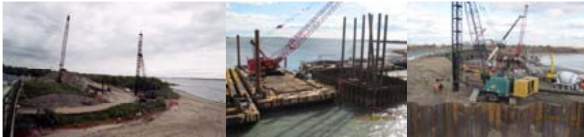
Paerdegat Basin Bridge in August 2010: The Installation of the New East Embankment for the Approach Roadway to the New Eastbound Bridge. November 2010: The Installation of New Piles at the New Waterway Pier Location. The New Eastbound Bridge Under Construction. The Photograph was Taken From the Future West Abutment and Shows the Pile Driving Equipment Mobilizing for the Installation of the Abutment Piles, the Placement of Concrete in the Piles at a New Pier Location, the Installation of New Piles at the New Waterway Pier Location, and the Temporary Work Trestle.
