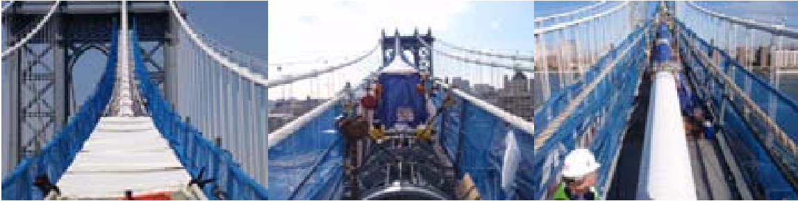
August 2010: Main Cable Work Platform With Containment Tarps. September 2010: View of Cable C With Wrapping Machine. October and November 2010: New Cable Guard Installed on Cable C.
