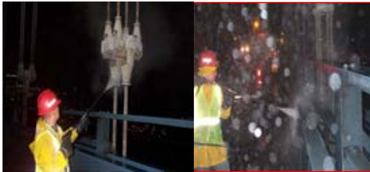
Power Washing the Corrosive Deicing Solvents Within the Range of the Roadway Splash Zone on The Manhattan Bridge in October 2007. Particular Attention is Directed to Cleaning the Gusset Plate. (Credit: Albert Hong)
