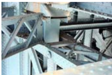
Truss Bearing on Manhattan Bridge. (Credit: NYSDOT)
