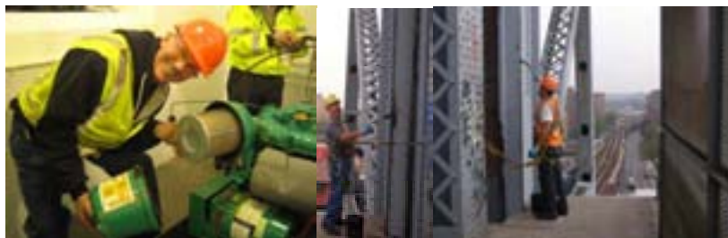
Oiler Tom Strommen Maintaining the Hydraulic Power Unit at the Hamilton Avenue Bridge in February 2010. (Credit: Vera Ovetskaya) Cleaning and Lubricating the Broadway Bridge. (Credit: Reza Taheri)
