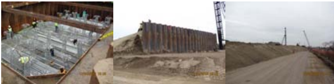
Paerdegat Basin Bridge in November 2010: The Installation of Steel Reinforcement for the New Pier Piles and Footing. The Installation of Steel Sheet and Piles at the New Bridge Abutment. The New West Embankment for the Approach Roadway to the New Eastbound Bridge. (Credit: Eric Callender)
