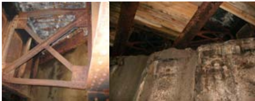
Deteriorated Bridge Deck With Exposed Rebar and Warped Steel Bracing Due to the Heat From the Fire. Timber Shielding on the Underside of the Bridge.
