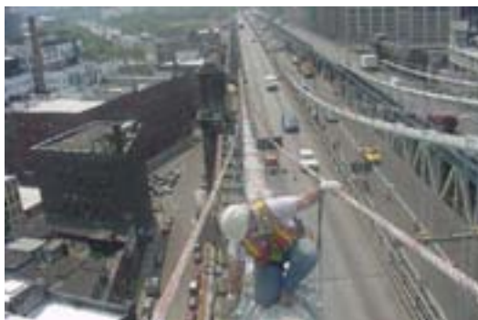
Inspector on Manhattan Bridge Cable. (Credit: NYSDOT)
