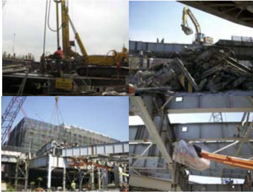
January 2010: Installing Caissons at the First Avenue On-Ramp. April 2010: Roadway and Steel Structure Demolition. Removal of Lead Based Paint From Structural Steel Cutline Locations Within a Class 3P Containment.
