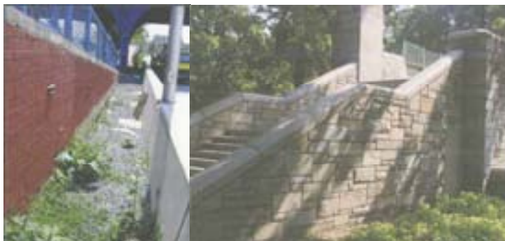
East Approach Cladding on the East 174 th Street Bridge. Abutment Wingwall Cladding on the West 173 rd Street Bridge.
