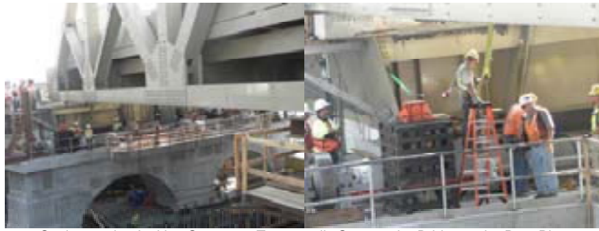
Setting up the Jacking System to Temporarily Support the Bridge at the Rest Pier. (Credit: Thomas Whitehouse)
