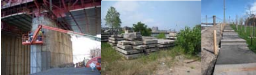
Removing the Roosevelt Island Bridge Panels. Piled Panels Awaiting Transfer to the Park.
