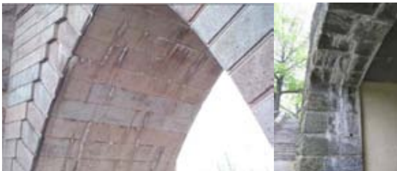
Moderate Efflorescence on the Brooklyn Bridge Brooklyn Tower North Gothic Arch in 2004. (Credit: NYSDOT) Efflorescence on the Underside of the Masonry Stones on the End Abutment of the Margaret Corbin Drive Bridge over Pedestrian Path Near Café.
