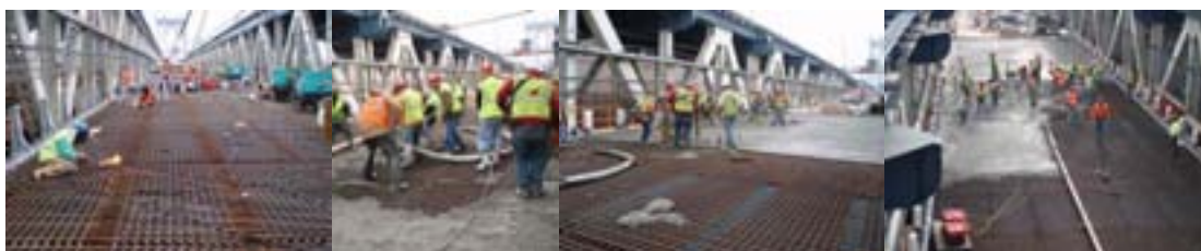
Installation of Full Width Grid Deck Panels on the Manhattan Bridge Lower Roadway in 2006. Pouring the Concrete.
