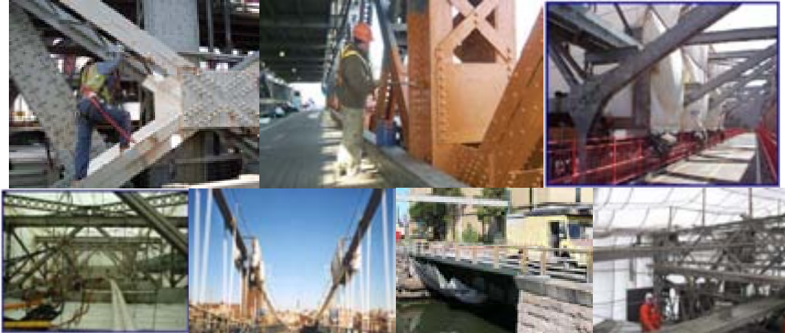
Williamsburg Bridge in June 2010: Application of Finish Coat at North Truss Diagonal. Salt Splash Painting on the Williamsburg Bridge. (Salt Splash Credit: Fouad Althaibani) Containment Examples. Manhattan Bridge - Painting Containment Structures on the Cables of the Manhattan Approach Span. Preventing Paint From Falling Into the Dutch Kills under the Hunters Point Avenue Bridge. (Credit: Sergiy Parayev) Working Inside the Queensboro Bridge Containment.
