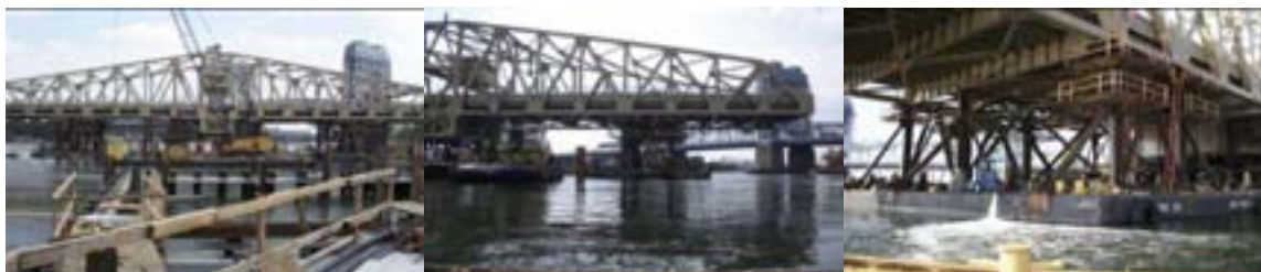
August 2010: Ballasting of Barges and Transferring the Swing Span From Twin Barge to Two Single Barges.
