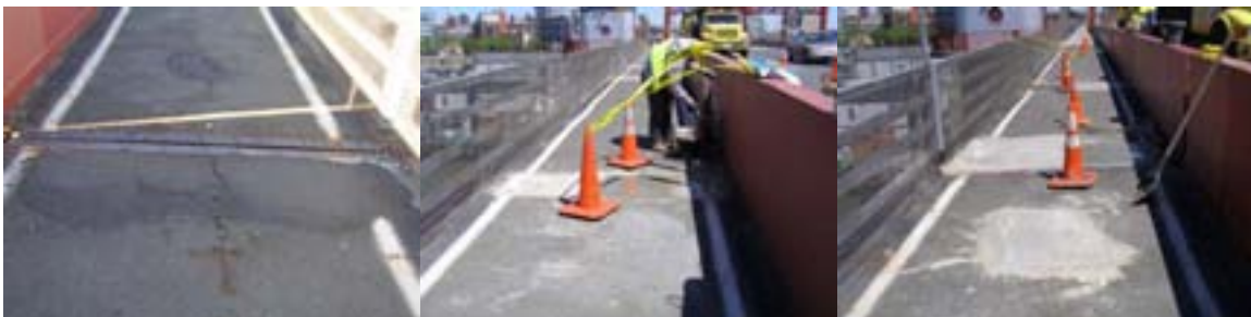
April 2010: Repairing Spalled Asphalt (a Tripping Condition) Near a Finger Joint on the Pulaski Bridge. (Credit: Samuel Teaw)
