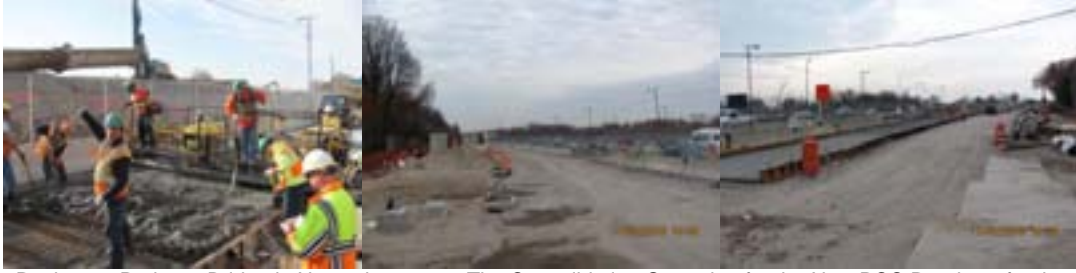
Rockaway Parkway Bridge in November 2010: The Consolidation Operation for the New PCC Roadway for the Westbound Off Ramp. The Installation of New Concrete Curbing, Catch Basin and Electrical Facilities for the New Westbound Roadway. The Installation of Formwork in Advance of the Installation of the New Westbound Roadway. (Westbound Roadway Credit: Eric Callender)
