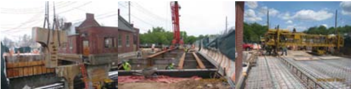
Annadale Road Bridge: Substructure Removal of Pier in Stage II in February 2010. Structural Steel Removal of Stringer in May 2010. Finishing Machine Used in Dry Run in June 2010.
