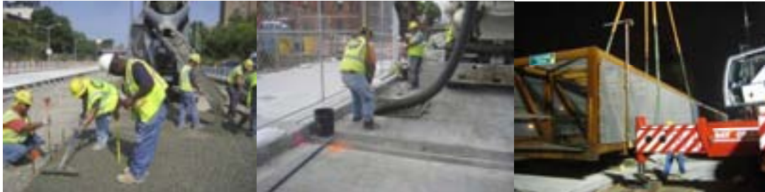
August 2010: Placing Concrete on the Northbound Left Lane. Cleaning the Drainage Structures in the Northbound and Southbound Approaches. Removed the Temporary Pedestrian Bridge, Allowing Pedestrians to Access the South Sidewalk of the New Bridge.
