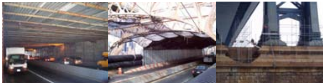
2007: Queensboro Bridge Lower Level and Upper Level Shielding. 2006: Erecting Scaffold to Build Painting Containment at Base of Brooklyn Tower of the Manhattan Bridge.
