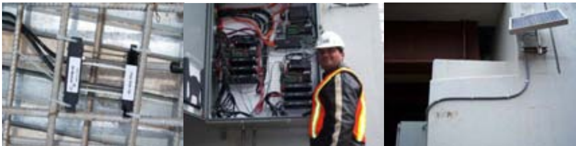
CPMP (Corrosion Penetration Monitoring Probe) Unit Installed on Clad Reinforcing Bars. Data Box and the Solar Panel.
