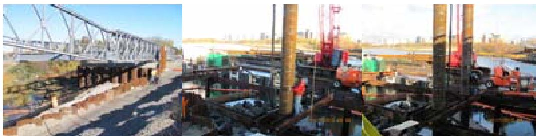
Fresh Creek Bridge in November 2010: The Temporary Bridge Superstructure Extending From the Temporary Bridge Abutment, the Temporary Steel Sheeting in the Foreground and in Front of the Abutment, and the Erosion and Sedimentation Controls Located Along the Perimeter of the Site and Water Body. Close up of the Installation of the Temporary Taper Tube Steel Piles via Barge-Mounted Crane. The Temporary Bridge can be Seen in the Background.
