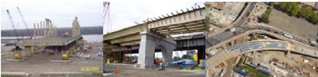
October 2009: Assembling the Willis Avenue Bridge Swing Span near Albany, New York. Willis Avenue Bridge August 2009: Installation of Tub Girders on Temporary Supports. September 2009: Existing and New Ramps to Bruckner Boulevard.
