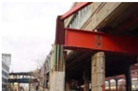
Queensboro Bridge Bent Column Ready for Jacking in 2005.
