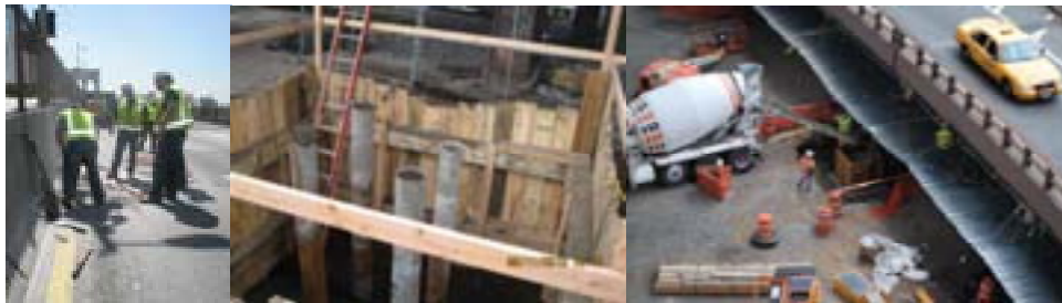
May 2010: Test Pit on Brooklyn-Bound Manhattan Approach. June and July 2010: Excavation and Concrete Placement for Pile Cap at Ramp A Bent 7A.
