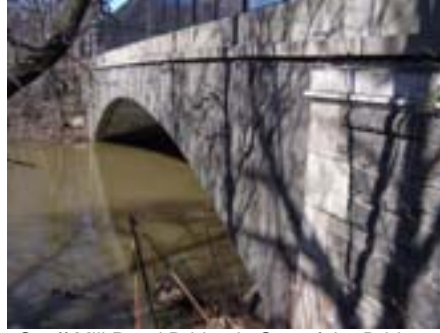
Snuff Mill Road Bridge is One of the Bridges Investigated for Scour Vulnerability and Found to be Structurally Sound, But it Remains Under Surveillance During Heavy Rains and Floods.
