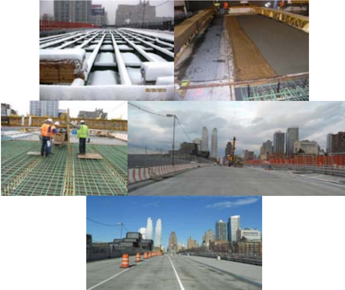
11 th Avenue Viaduct: Demolition of the Old Deck in February 2010. Inspecting Machine Setup Prior to Placing the New Deck Slab Concrete in October 2010. First Concrete Pour in August 2010. (Credit: Hui Yang) Working on Bridge Rail and Pedestrian Fencing in November 2010. (2 nd Rail Credit: Hui Yang)
