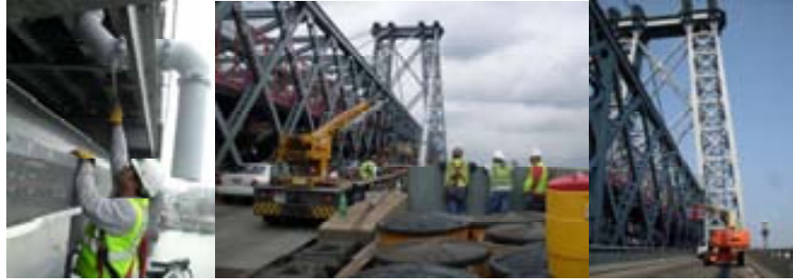
May 2010: Looking East at the Application of the Intermediate Coat on the South Outer Roadway Downspout Between PP50W and PP51W. June 2010: Looking East at the Replacement of the One Rail Bridge Rail at the Manhattan End Span. June 2010: Looking West at the Touch-Up Painting of North Truss at Brooklyn End Span.
