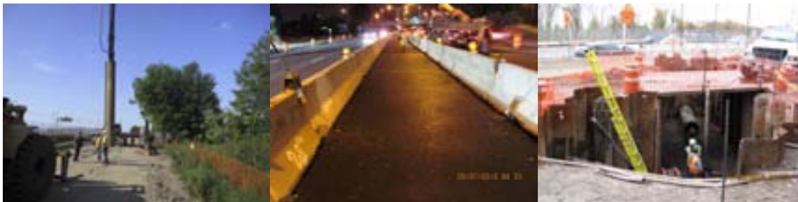
Fresh Creek Bridge in July 2010: Installing Sheathing Along the Southwest Area of the Shoreline. The Nighttime Installation of Temporary Asphalt Pavement in the Median of the Belt Parkway. November 2010: The Installation of the New Ductile Iron Sludge Force Main Being Installed Through a Jacking Sleeve that Crosses Under the Existing Roadway. (Sludge Force Main Credit: Eric Callender)
