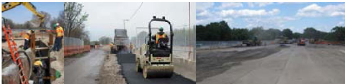
Paerdegat Basin Bridge in April 2010: The New Ductile Iron Sludge Force Main Being Installed in a Trench. The Placement and Rolling of Temporary Asphalt for the Temporary Pedestrian/Bicycle Path. June 2010: The Grading in Advance of the Placement of Embankment Material on the Eastern Approach to the New Bridge.
