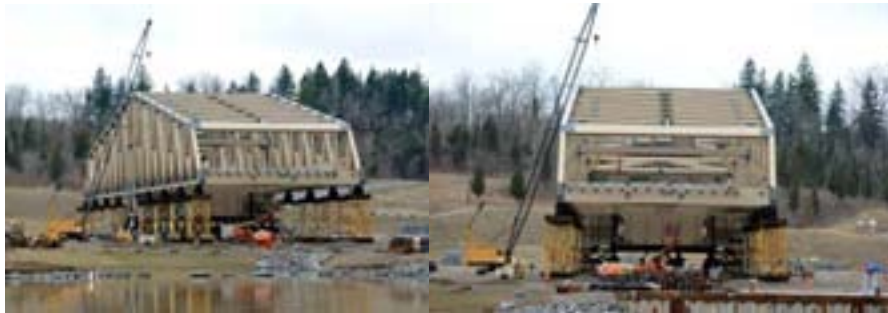
Late March 2010: Assembling the Willis Avenue Bridge Swing Span near Albany, New York. (Credit: Bernard Ente)
