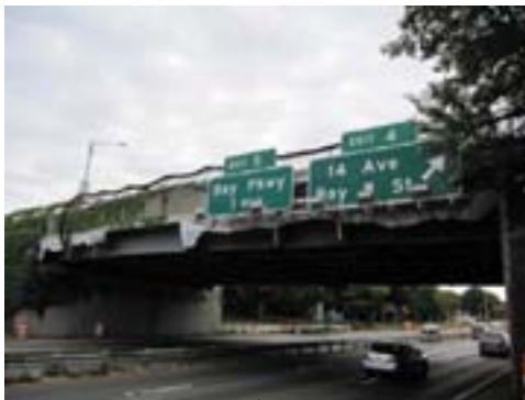
Contract Painting of Bay 8 th Street over Belt Parkway in August 2010. All Abrasive Blasting Activities Were Conducted During the Nightshift. Prior to the Abrasive Blasting Operation the Environmental Inspector Conducted Air Flow Measurements and Measured the Negative Pressure Inside of the Class 1A Containment System.
