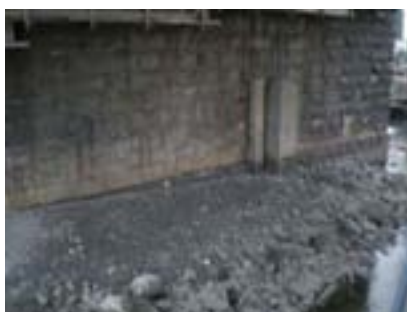
Eroded Riprap Pier Protection at Pier 11 of Old Willis Avenue Bridge in 2008. (Credit: NYSDOT)
