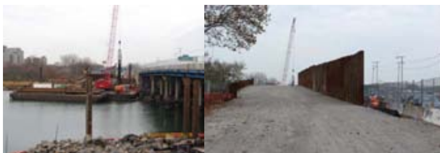
Fresh Creek Bridge in November 2010: The Installation of the Temporary Taper Tube Steel Piles via a Barge-Mounted Crane. The Piles are Designed and Installed to Support the Temporary Bridge. The Temporary Approach Roadway to the Temporary Bridge. (Credit: Eric Callender)
