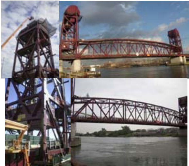
January 2010: Delivering Machinery Components to the East and West Machinery Rooms. February 2010: Removing Railing From the Roosevelt Island Side of the Bridge. July 2010: Cleaning and Dismantling of the Platform Under the Main Span.
