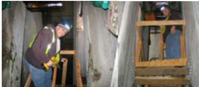
Carpenter John Green Installing a Platform for Strain Gauge Measurement at the Hamilton Avenue Bridge in March 2010. (Credit: Vera Ovetskaya)
