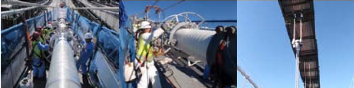
October and November 2010: New Cable Guard Installed on Cable C. November 2010: New Suspender Installed on Main Cable C.
