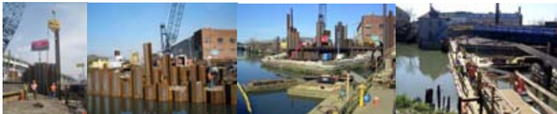
Sheet Piling of Cofferdam. Closeup of Sheet Pile Driving Operation for the West Abutment. (West Abutment Credit: Reza Lotfi) Reconstruction of West Abutment of the Borden Avenue Bridge in April 2009. (Credit: Bernard Ente)
