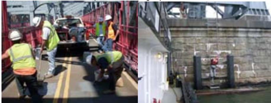
May 2009: Looking West at the Repair of the North Footwalk Overlay between PP10W and PP11W. August 2009: Looking North at Installation of the Fender System at the Manhattan Main Tower.
