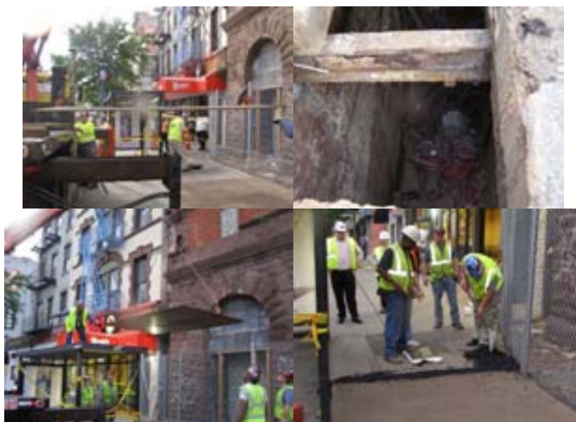
Bridge Repairer and Riveter Joseph Hickey Operating a Boom Truck Hoisting a Plate, While Executive Director of Bridge Preventive Maintenance and Repair Thomas Whitehouse (in the Background) Dumps Bags of Cold Patch. The Exposed Vault. Bridge Repairer and Riveter Chris Mauldin Atop the Bus Shelter Guiding the Placement of the Steel Plate; Executive Director of Bridge Preventive Maintenance and Repair Thomas Whitehouse and Bridge Repairer and Riveter Scott Mahaffey (Behind the Shelter); Bridge Repairer and Riveter James Wright III and Supervisor Bridge Repairer and Riveter Gean Pilipiak; and Bridge Repairer and Riveter Joseph Hickey (Obscured). EDC Representatives (Back Row); EDC's Emergency When and Where Contractor Laborer and Supervisor (Front Left); Supervisor Bridge Repairer and Riveter Gean Pilipiak (Middle); and Executive Director of Bridge Preventive Maintenance and Repair Thomas Whitehouse Leveling the Cold Patch to Set the Steel Plate. (Credit: Reza Taheri)
