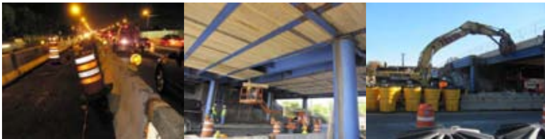
Rockaway Parkway Bridge in July 2010: The Nighttime Installation of Temporary Asphalt Pavement in the Median of the Belt Parkway. September 2010: Installing Planks Along the Lower Flanges of the Stringers. November 2010: Stage II Demolition of the Existing Bridge Superstructure.
