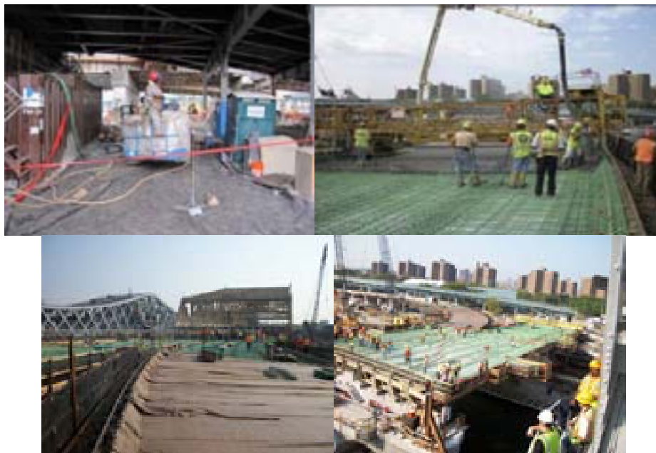
August 2010: Removal of Lead Based Paint From Structural Steel Cutline Locations Within a Class 3P Containment at the Manhattan End Span. Concrete Placement for Decks at Spans A10, A11, and 3.
