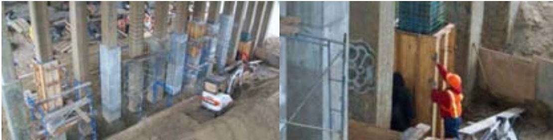
Pier 3 Column Repair in December 2008. (Credit: NYSDOT)
