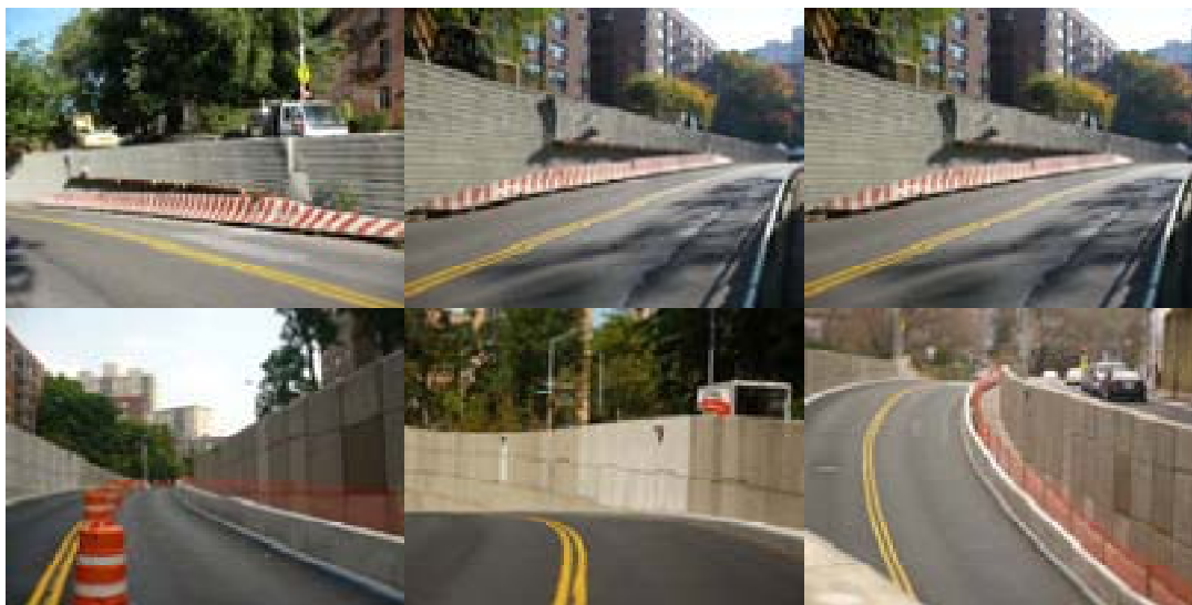
Kappock Street Retaining Wall in Riverdale, Before and After Repairs. The Existing 300-Foot Long Parallel Concrete Roadway Retaining Walls on Both Sides of Kappock Street Were Deteriorated and Leaning, and Were Replaced with New Modular Retaining Walls in the Summer of 2009.
