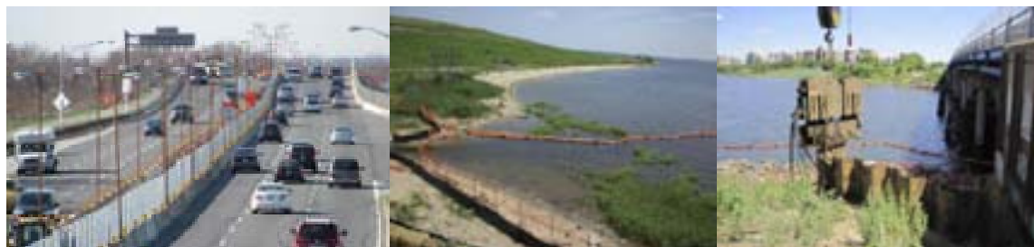
Fresh Creek Bridge in March 2010: The Temporary Lighting System Installed on the Temporary Median Barrier Leading up the Eastern Approach to the Bridge. May 2010: Turbidity Curtain Along the Shoreline. June 2010: Equipment for Driving in Sheet Metal Piling.
