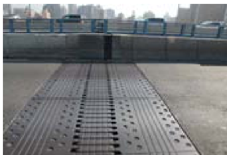
Manhattan Bridge Finger Dam. (Credit: Jagtar Khinda)
