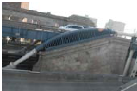
Manhattan Bridge Saddle. (Credit: Jagtar Khinda)
