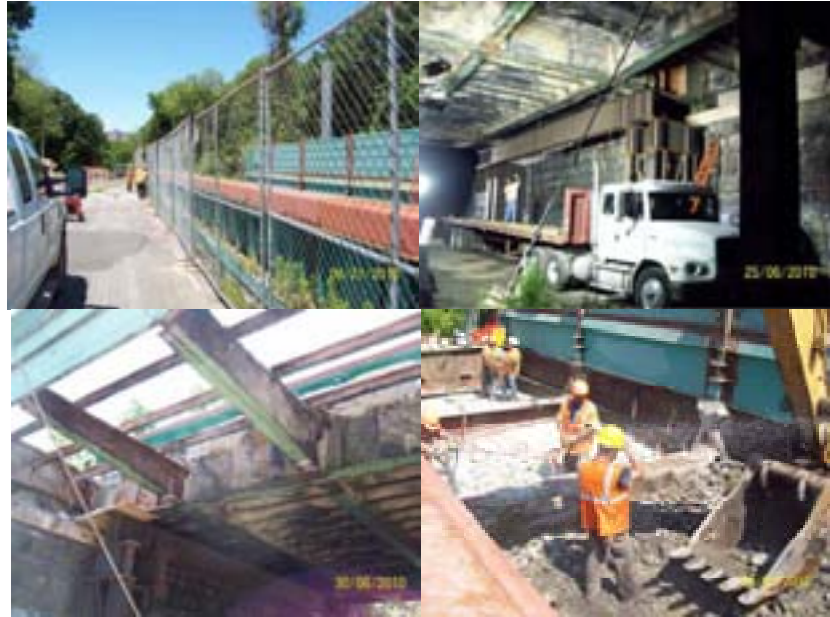
Shore Road Circle Bridge: Preparation of MPT and Work Zone, Installation of Temporary Shoring Towers, and Partial Steel Removal in June 2010.
