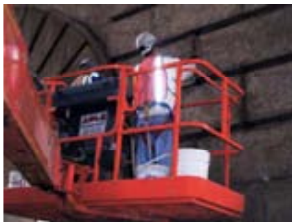
Pointing Joints on the East Face of the Brooklyn Anchorage of the Manhattan Bridge.
