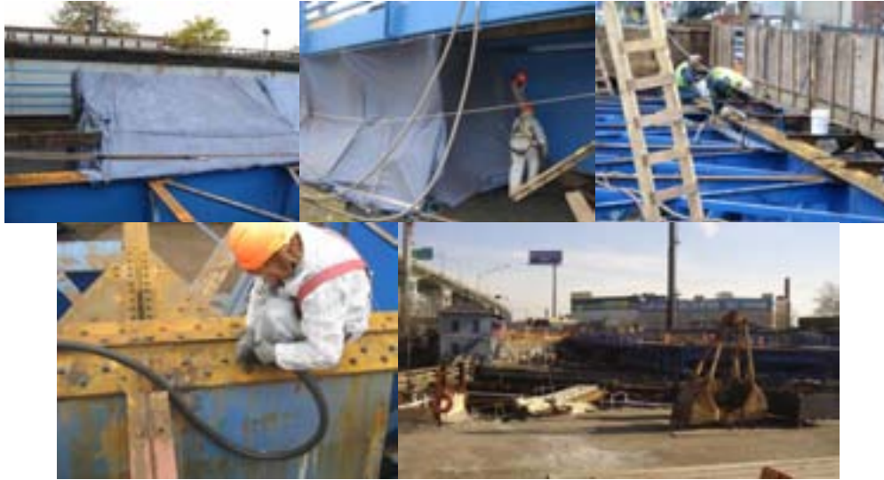
October and November 2009: Paint Removal with Vacuum Shrouded Power Hand Tool Under a Class 3P Containment. Ironworkers Removing Rivets and Dismantling Steel. December 2009. (Credit: NYSDOT)
