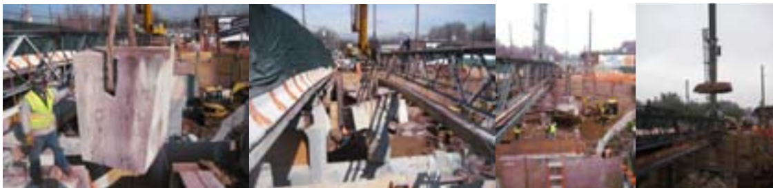
Annadale Road Bridge: Removing the South Abutment and Center Pier in March 2009. : Removing the North Abutment Footing and the Partly Embedded Abandoned Sewer Pipe Containing Asbestos in May 2009.
