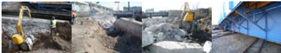
Demolition of the West Abutment and Wingwall in February 2009. (Third View Credit: Reza Lotfi) February 2009. (Credit: Tamara Berlyavsky)
