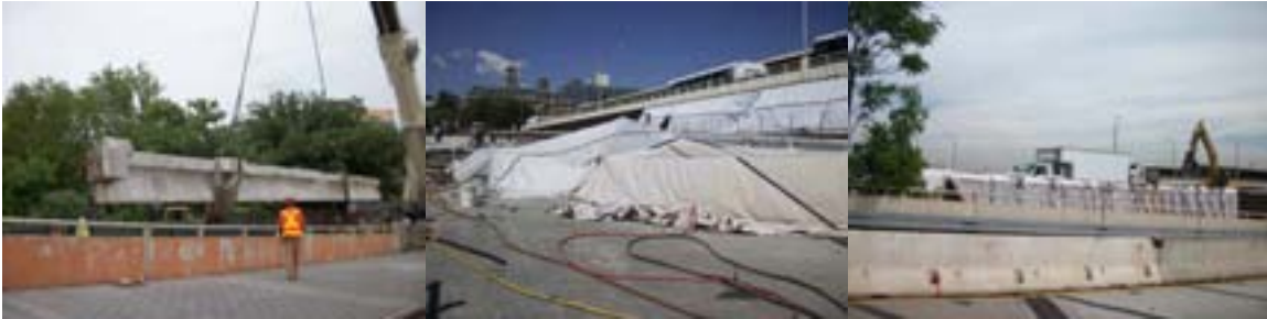
July 2010: Removing Concrete Support Beams From Ramp A. Preparing for Power Hand-Tool Operation at Ramp D. Class 3P Containment at Ramp D.
