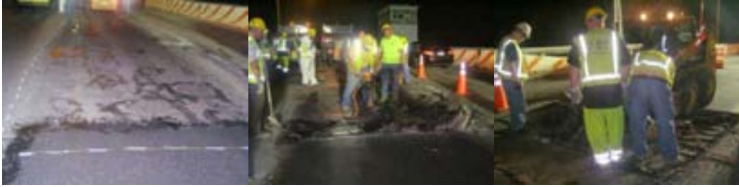
Resurfacing the Belt Parkway Bridge over Mill Basin on August 3, 2009. The Crew Completed a 13'x29' Cut in the Eastbound Center Lane, West Approach Spans. The Area Before Breakout, Exhibiting Rutting, Cracking and Excessive Patching. Breakout and Removal of Deteriorated Wearing Surface.
