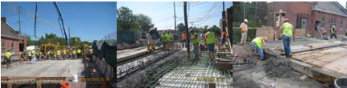
Annadale Road Bridge Stage II: Concrete Placement of the Deck Slab in June 2010 and of the Approach Slabs in July 2010.
