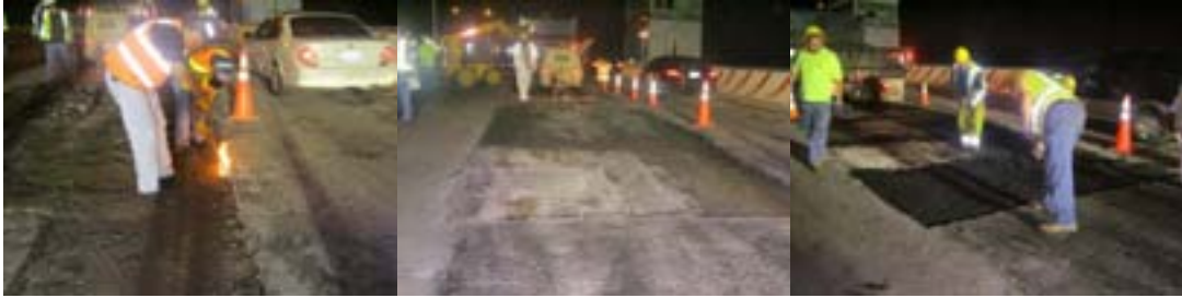
Belt Parkway Bridge over Mill Basin: Ironworker Assisting the Crew. Prepped Cut, Ready for Asphalt. Installation of New Asphalt. (Credit: Yousef Demis)
