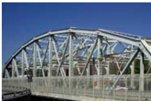
Macombs Dam Camelback Truss.
