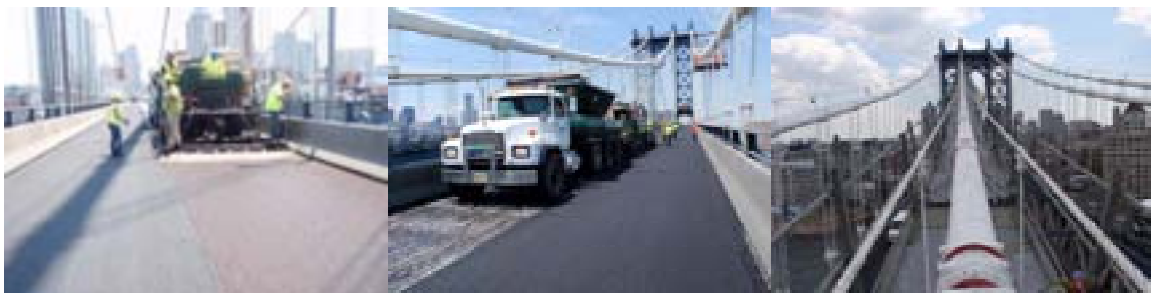
June 2010: Placement of Micro-Surfacing Layer on North Upper Roadway. July 2010: Main Cable Work Platform for Cable C.
