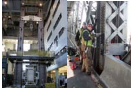
2009: Testing the Intermediate Tower Bearings at Lehigh University in January 2009. March 2009: Looking East at the Bolting up of the Truss Reinforcement at PP10W in Preparation for Bearing Replacement.
