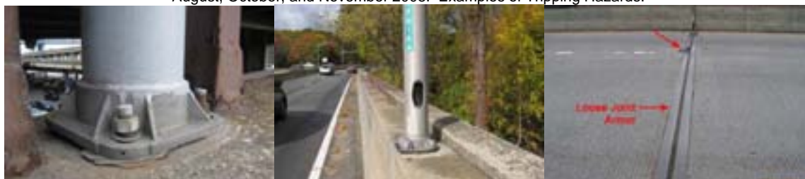
February 2008: Loose Bolts at the Lighting Base. October 2008: Electrical Hazard, and Loose Joint.
