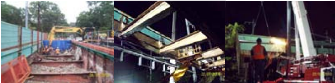
Shore Road Circle Bridge: Clearing Structural Steel for Demolition and Disassembling Steel Members in July 2010.
