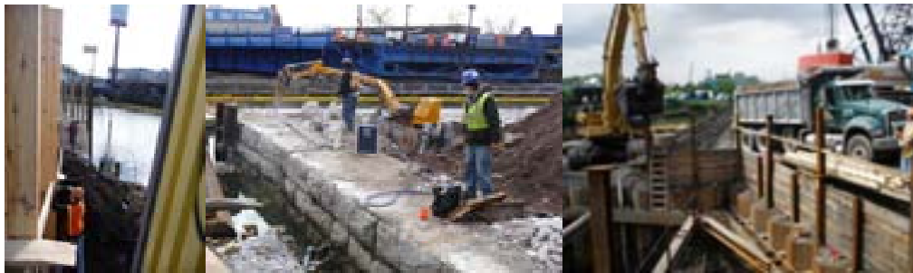
Borden Avenue Bridge in March 2009. (Credit: Tamara Berlyavsky) Demolition and Disposal of West Abutment Wall. (Credit: Reza Lotfi)
