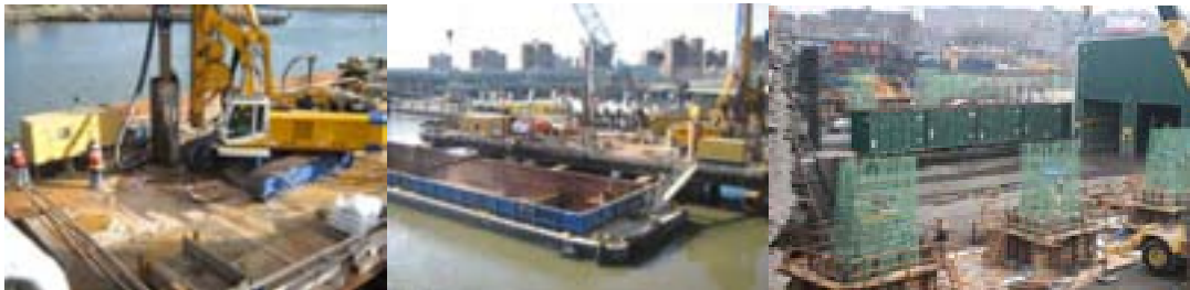
2009: The Primary Equipment Utilized During Caisson Installation was an Augering System Driven Into the River Bottom. Water From the Harlem River was Pumped Into the Augering System. All Augered Waste was Pumped out of the Caisson Into a Weir Barge. All of the Water Within the Weir Barge was Filtered Through a Fabric Medium and Pumped Back into the Harlem River. This System Effectively Removed all of the Solids From the Wastewater. April 2009: Willis Avenue Bridge Pier 9 Rebar Columns.
