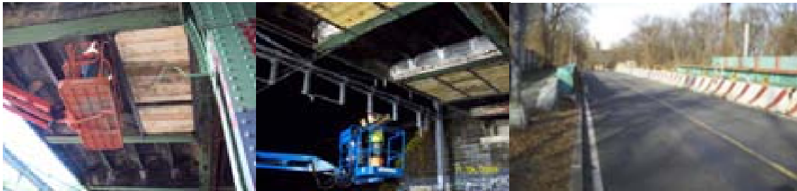
Shore Road Circle Bridge: Installing a Reinforcing Timber Beam Underneath the Existing Floor-Beam in Preparation for Stage 1A Construction in June 2009. Installing the Demolition Shielding Over Track #1 for Stage 1A in November 2009. Left Roadway in December 2009. (December Credit: NYSDOT)
