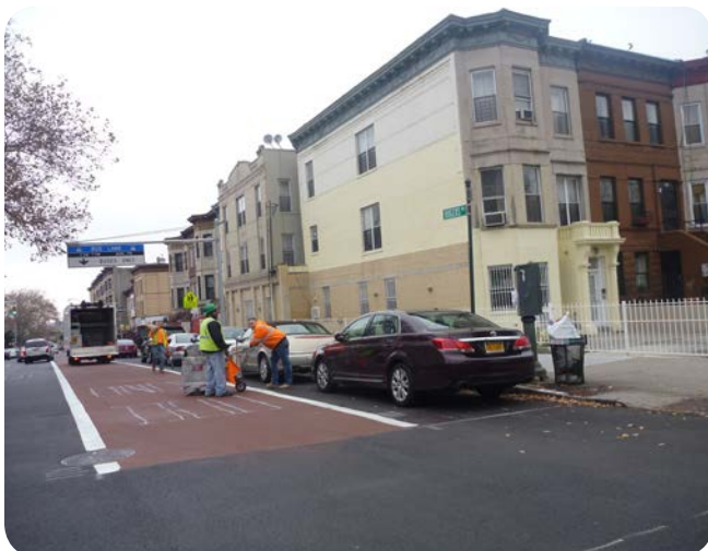
Bus lane painting on Rogers Avenue
