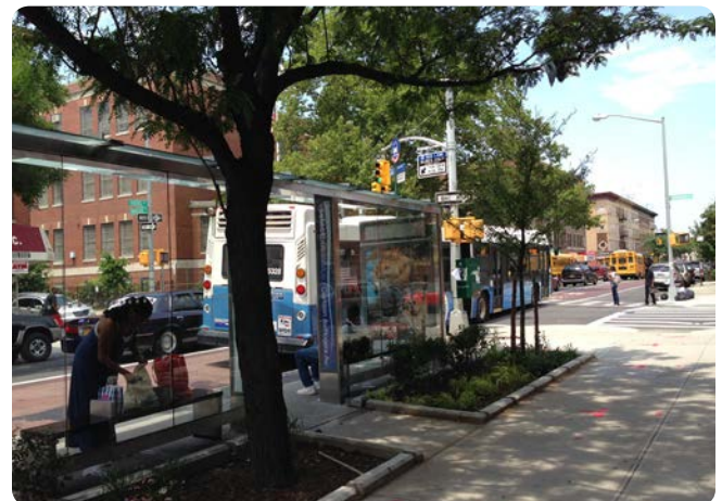
Bus bulb station at Nostrand Avenue and Parkside Avenue with shelter and added greenery
