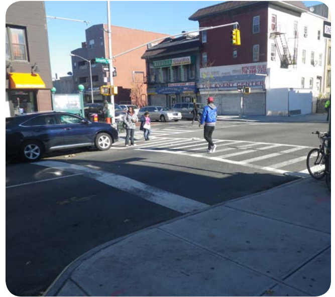
Neckdown on Lafayette Avenue at Nostrand Avenue (SW Corner)
