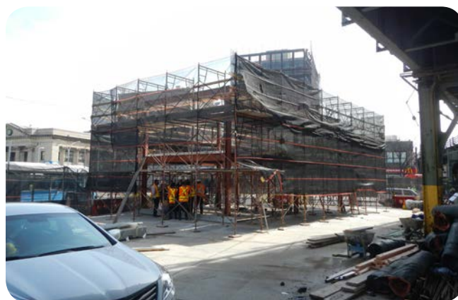
NYCT building under construction as of 03-2016
