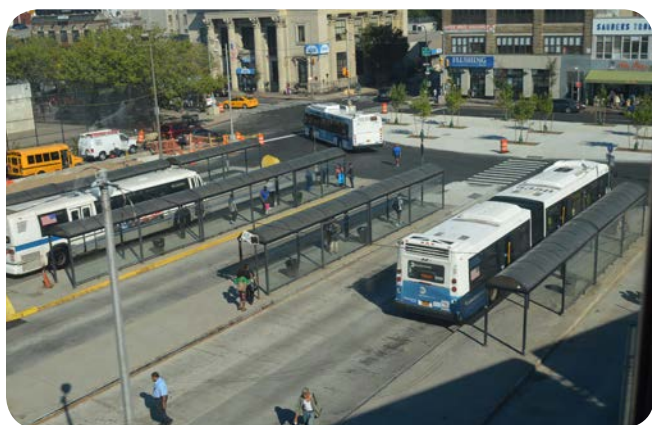
Williamsburg Bridge Bus Plaza Construction Progress as of 11-2015
