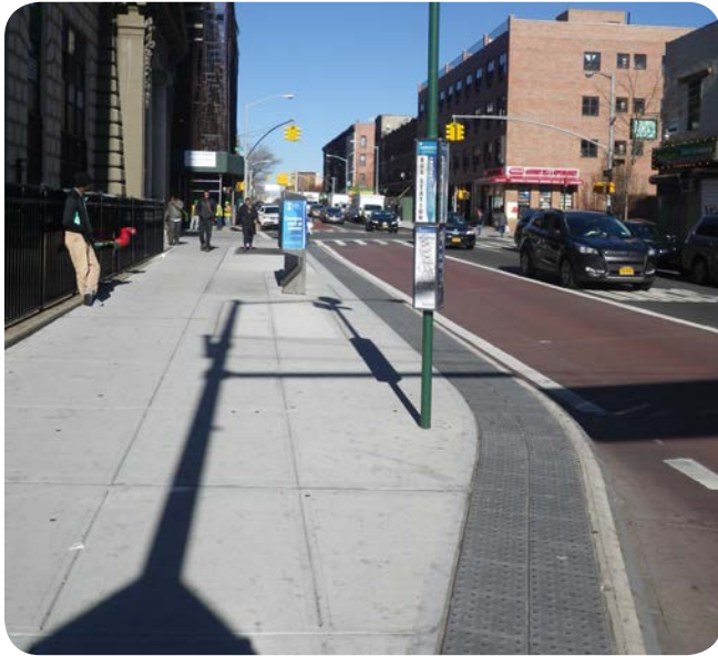
Bus Bulb on Nostrand Avenue at Gates Avenue (SW corner)
