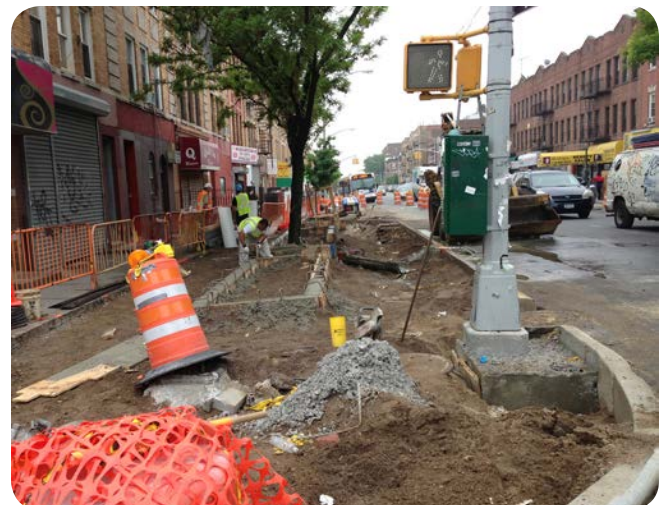
Bus bulb construction on Rogers Avenue at Parkside Avenue
