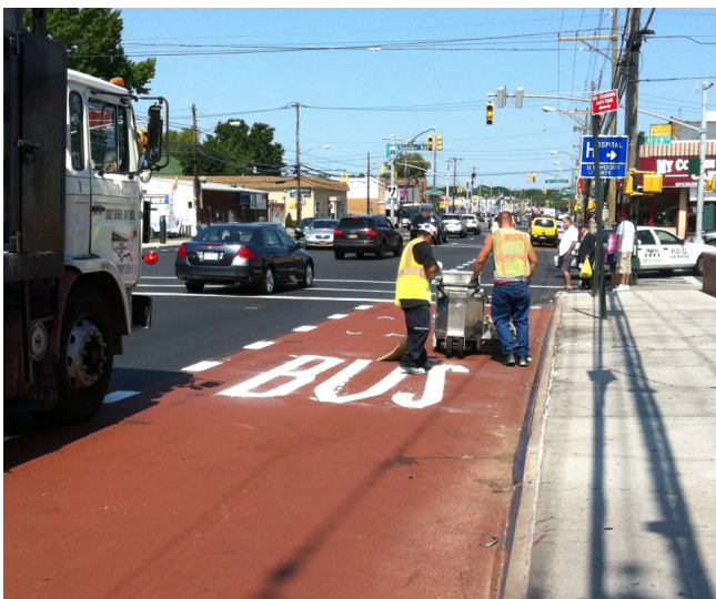
Figure 5 – Installation of bus lane on Hylan Blvd
