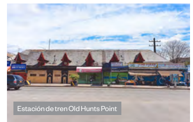
Corredor de Hunts Point Avenue
