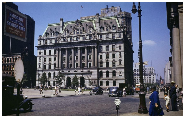
The Surrogate's Court, 31 Chambers Street, 1939. Credit: NYC Municipal Archives.
