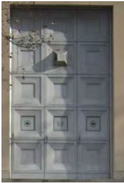
Cadman Plaza Door: Existing
