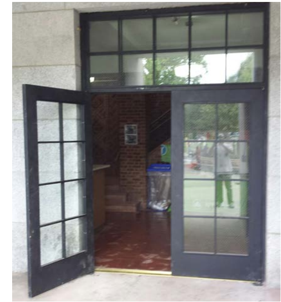
Williamsbridge Oval: Painted Steel with Divided Lights
