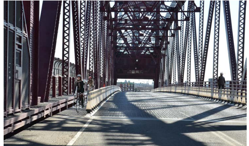
Existing configuration of Roosevelt Island Bridge - Facing east
