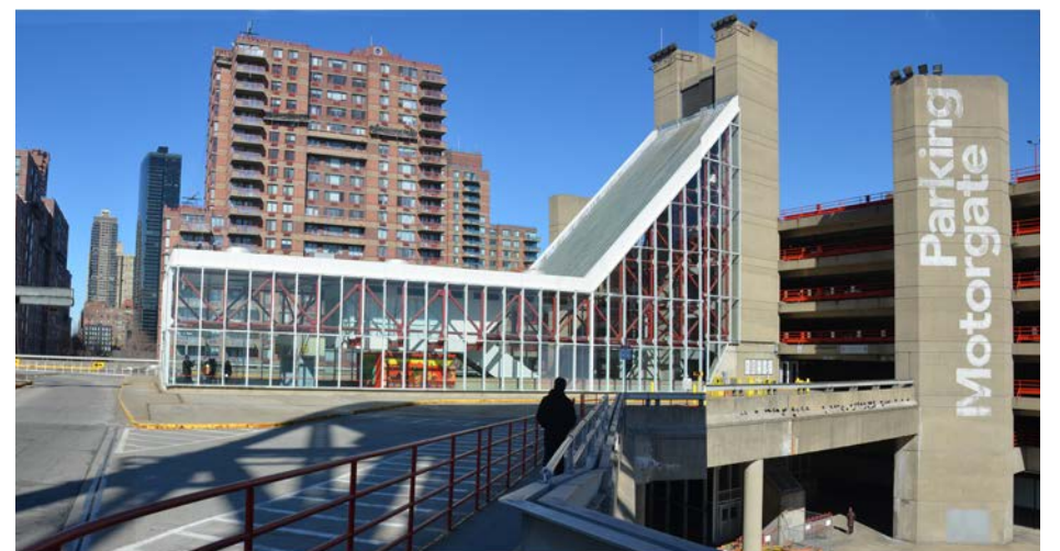
Existing Bike/Ped connection between RI Bridge and Motorgate
