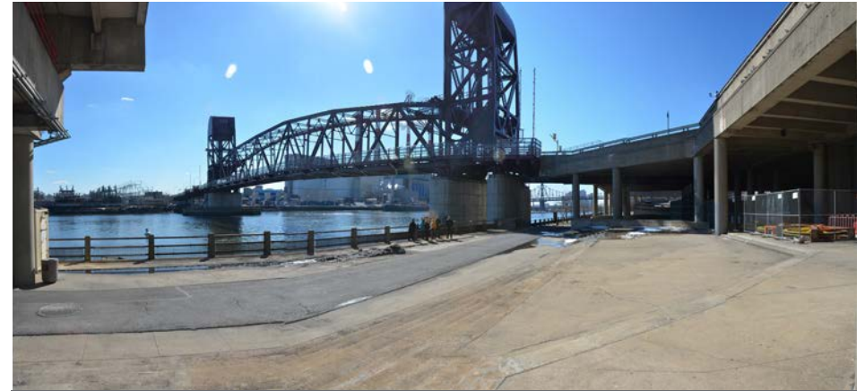
Existing connection to Roosevelt Island Greenway from Motorgate Garage
