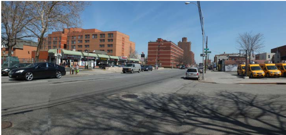
Existing Street Conditions of 21st Street at 33rd Road
