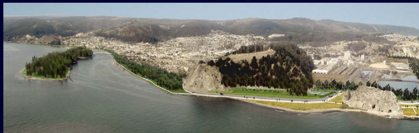
Credit: ELEMENTAL S.A.
