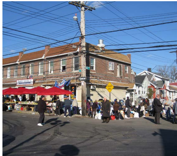
Rockaways, Queens following Hurricane Sandy
