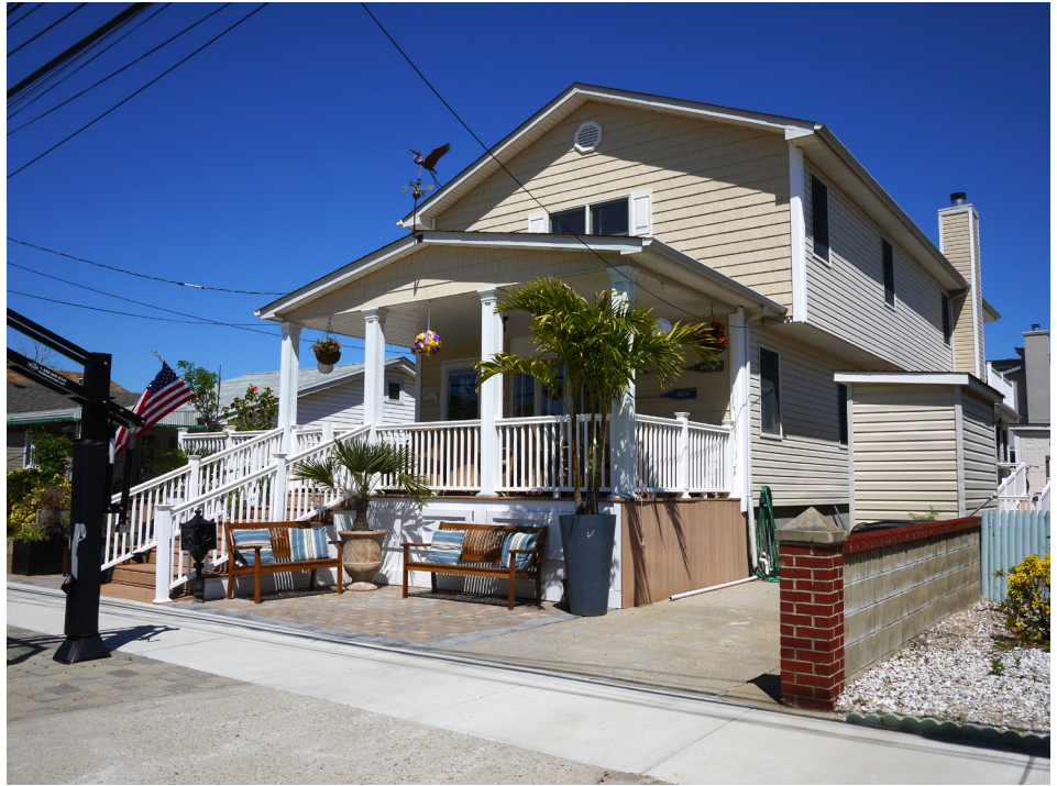
Elevated home in Breezy Point, Queens
