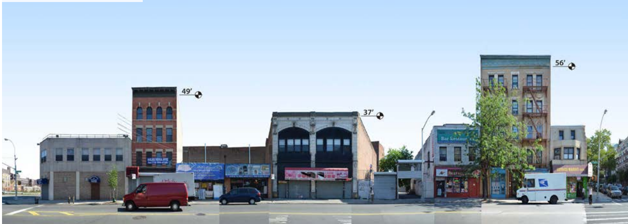
FIGURE 7 | Existing Conditions, northwest along East Tremont Avenue, half a block east of Tremont Station.
