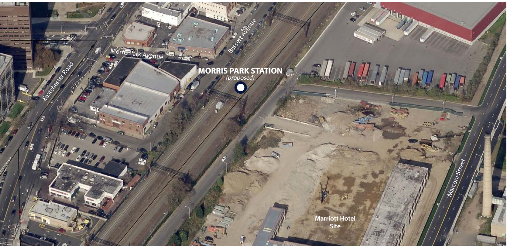
FIGURE 1 | Proposed entrance area to Morris Park Station, located where Morris Park Avenue meets Amtrak’s Hell Gate Line at Basset Avenue. The station would provide east-west pedestrian access over the rail which currently does not exist. Source: © 2011 Pictometry International Corp.
