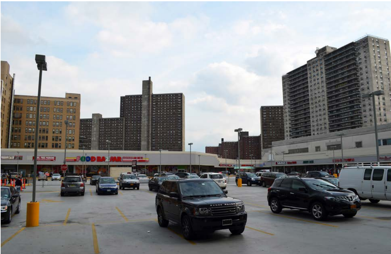
FIGURE 18 | Concourse Plaza, across the street from the Bronx Hall of Justice on East 161st Street. The low-scale buildings and large parking lot are largely out of context in the area, prioritizing automobile access to these amenities over pedestrian access
