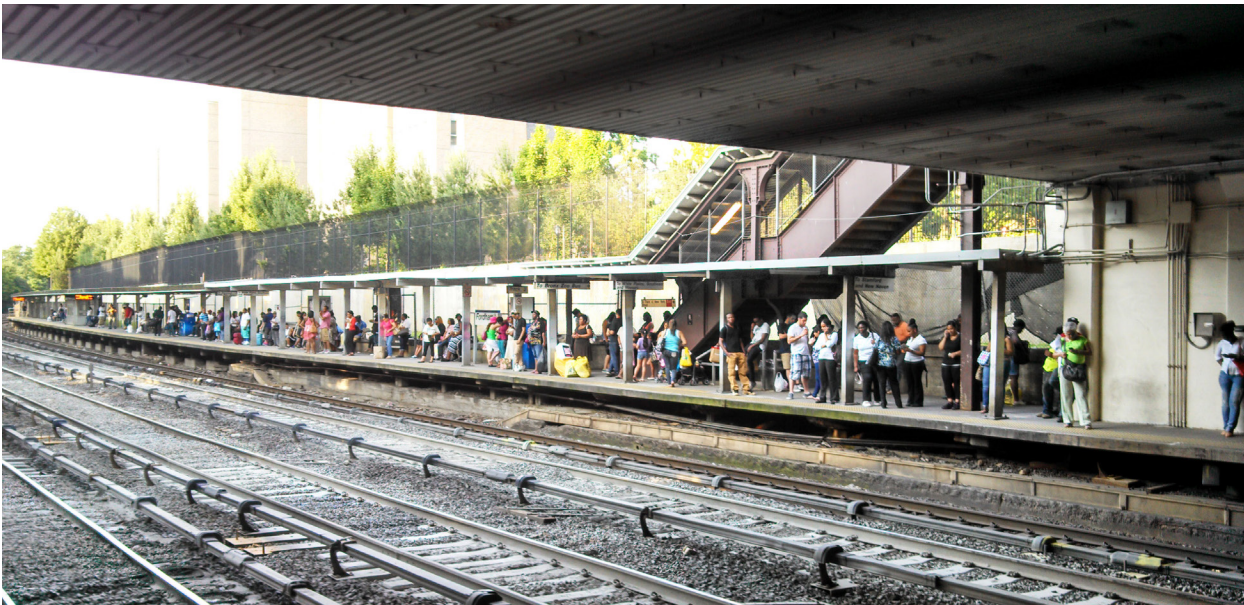
FIGURE 6 | Fordham Metro-North Station on the Harlem Line, one of the busiest stations in the system. Many Bronx residents depend on this public transportation option to commute to and from work.
