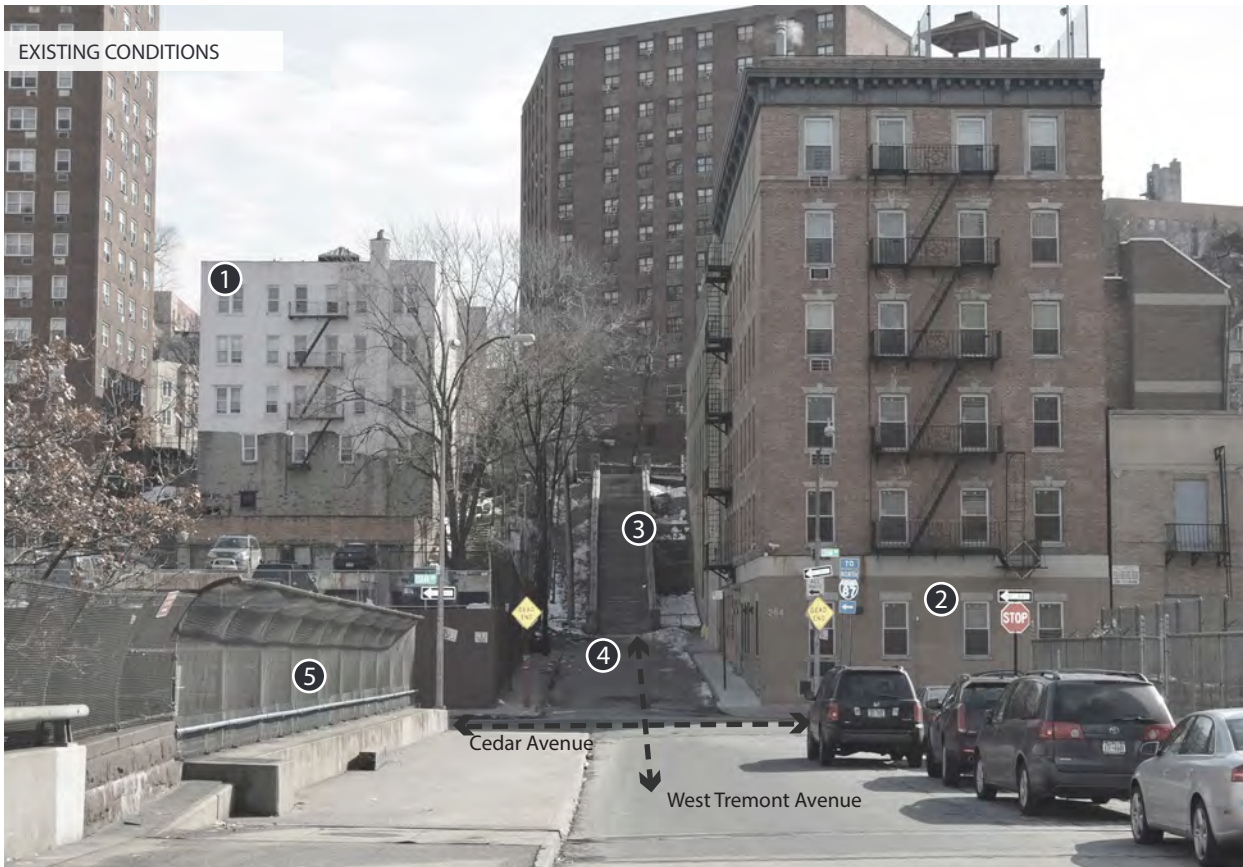
FIGURE 4 | Existing Conditions at Cedar Avenue and West Tremont Avenue
