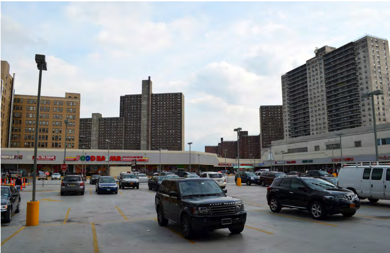
FIGURE 18 | Concourse Plaza, across the street from the Bronx Hall of Justice on East 161st Street. The low-scale buildings and large parking lot are largely out of context in the area, prioritizing automobile access to these amenities over pedestrian access
