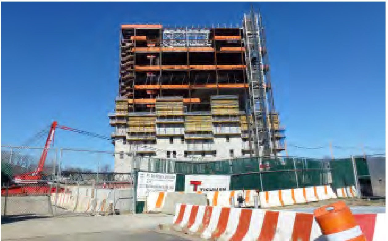
FIGURE 5 | The Public Safety Answering Center II (PSAC II), currently under construction. When it opens its doors in 2015, it will house approximately 850 employees.
