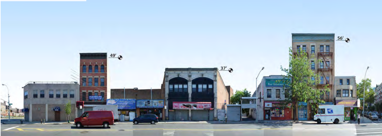
FIGURE 7 | Existing Conditions, northwest along East Tremont Avenue, half a block east of Tremont Station.
