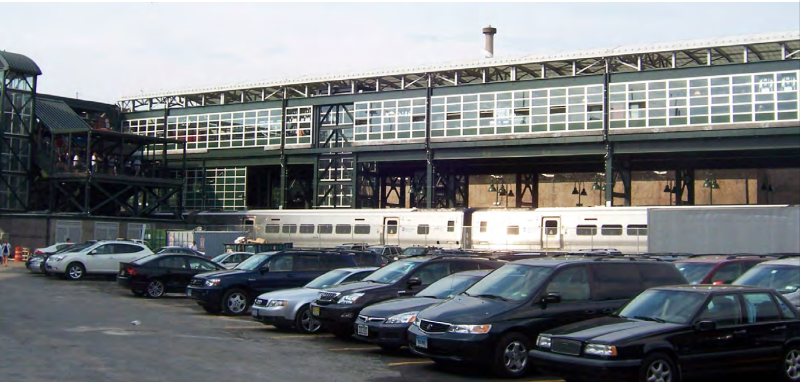
FIGURE 9 | Metro-North pedestrian bridge. In 2009, a Metro-North station opened at 153rd street to serve the new Yankees Stadium and the Highbridge neighborhood in the Bronx. The new station includes an enclosed pedestrian bridge that bypasses roadways and other pedestrian implements to ease pedestrian access from the station to the stadium and other destinations to the east. The sleek design and wide stairway entrances are inviting to pedestrians. The Arts for Transit mosaics which line the interior walls of the structure provide interest along the 450-foot corridor.
