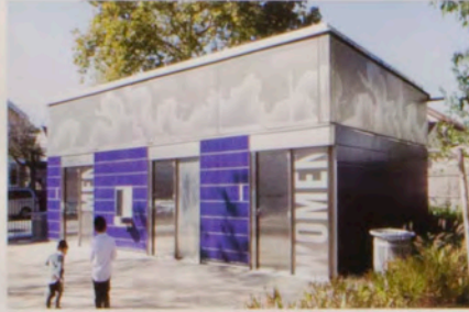
Lyons Square Bathroom
