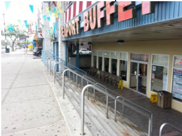
Below grade retail space in cellar
