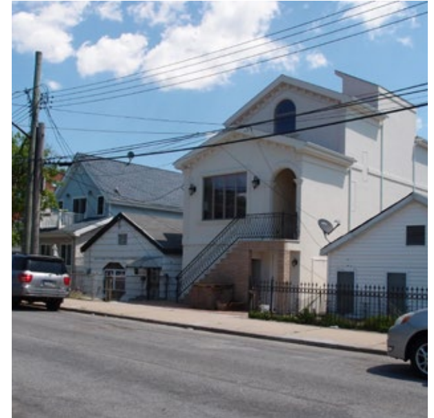
Former bungalow home retrofitted and elevated above the DFE
