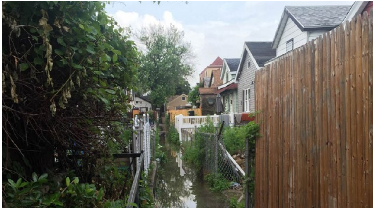
Flooding after regular rain event in Stanton Court
