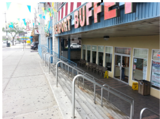
Below grade retail space in cellar
