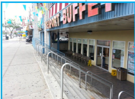
Below grade retail space in cellar
