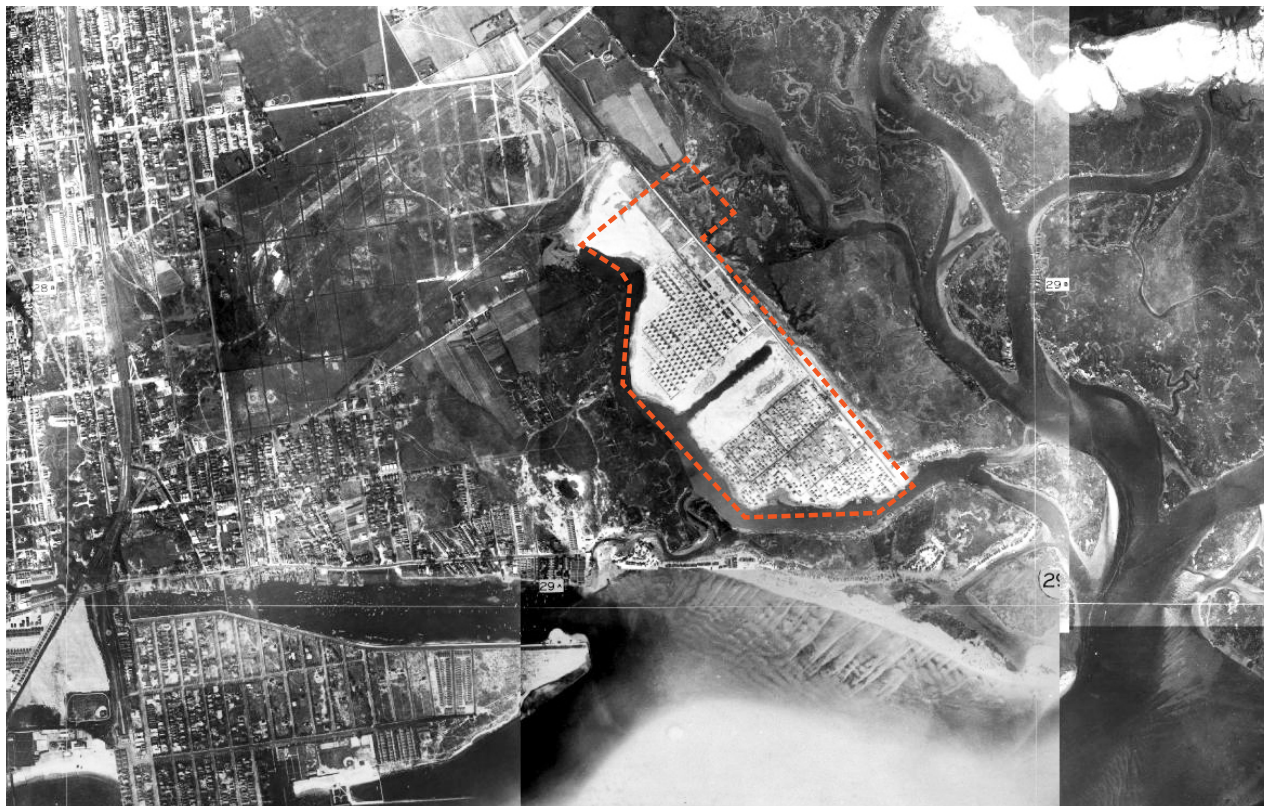
© 1924 Aerial Photography, New York City Department of Information Technology and Telecommunications.
