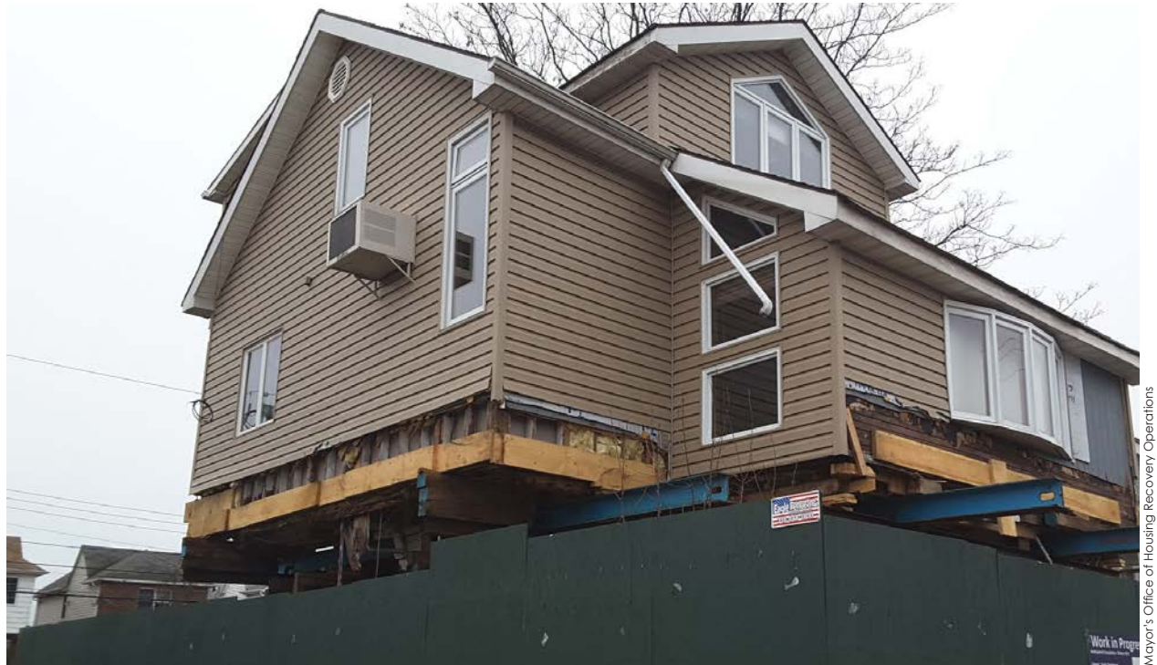
Build It Back home elevation in Gerritsen Beach
