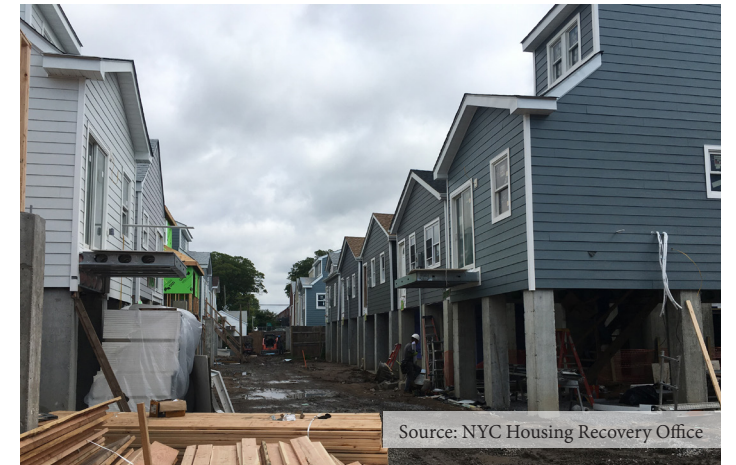
Home elevations and street reconstruction, Sheepshead Bay, Brooklyn
