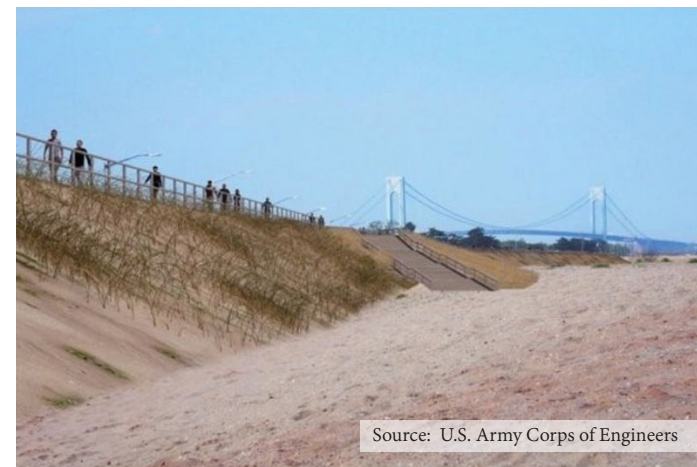
East Shore Seawall Project. Future Conditions: Buried Seawall with new elevated promenade, Midland Beach area looking north
