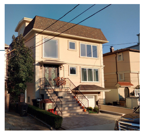
House retrofitted to comply with Appendix G in Bergen Beach, Brooklyn
