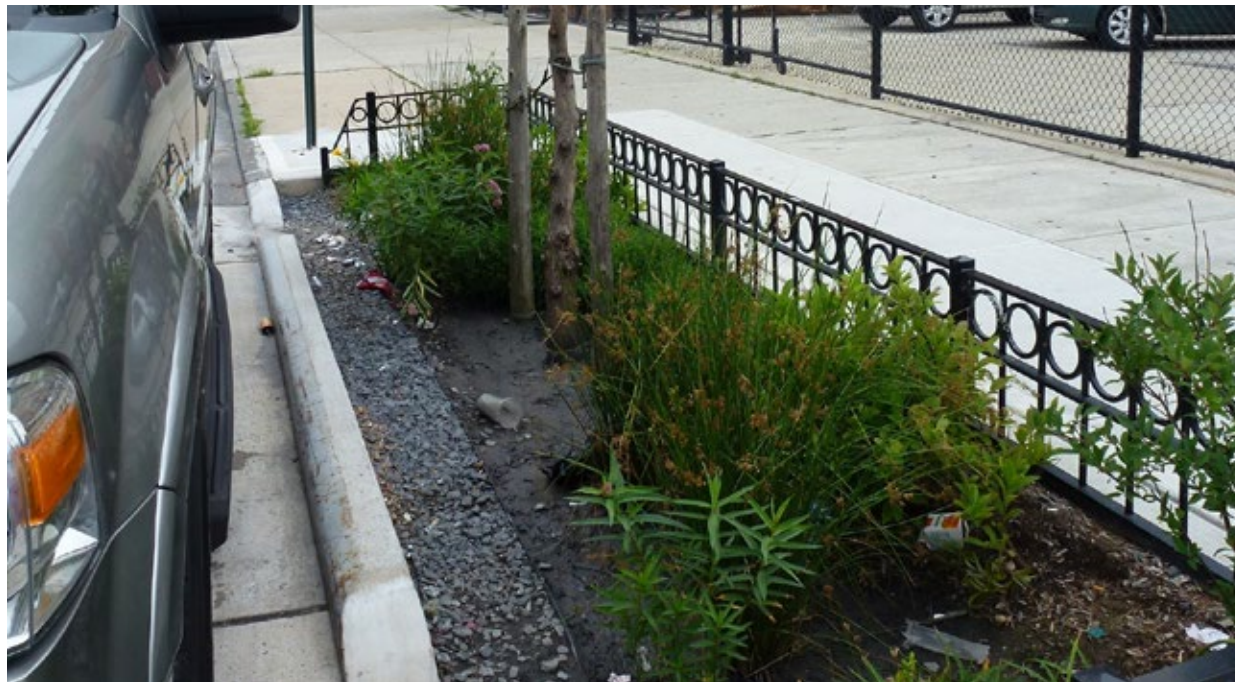
Right of Way Bioswale installed through NYC Green Infrastructure Program
