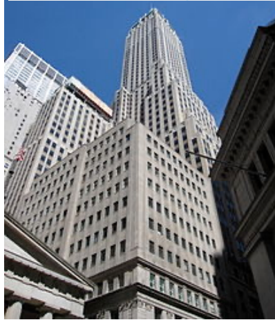
Office-to- daycare (40 Wall St - 2 floors)
