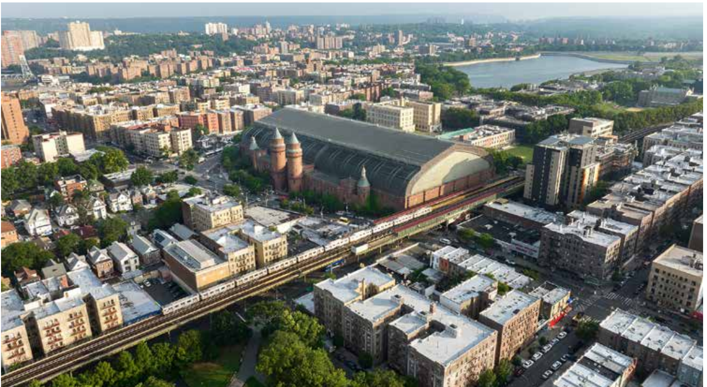
Kingsbridge Armory in The Bronx. Credit: NYCEDC
