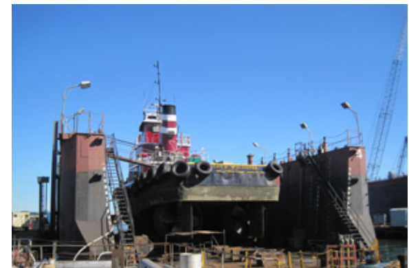
Tugboat repair at Caddell Dry Dock
