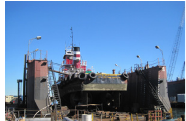
Tugboat repair at Caddell Dry Dock
