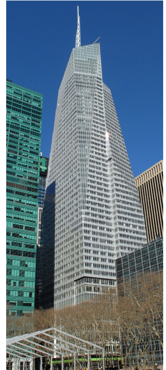
state-of-the-art office construction
