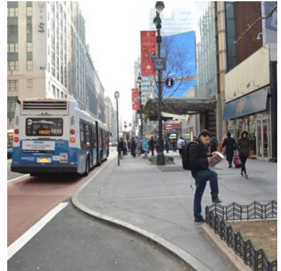
Bus bulbout at Seventh Avenue and West 34th Street
