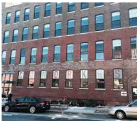
68 3rd Street, recently renovated for offices
