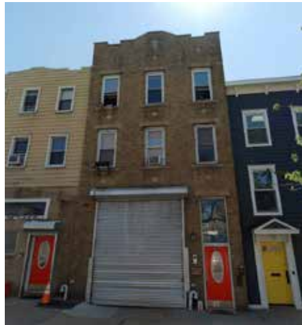
Existing residential use on Sackett Street
