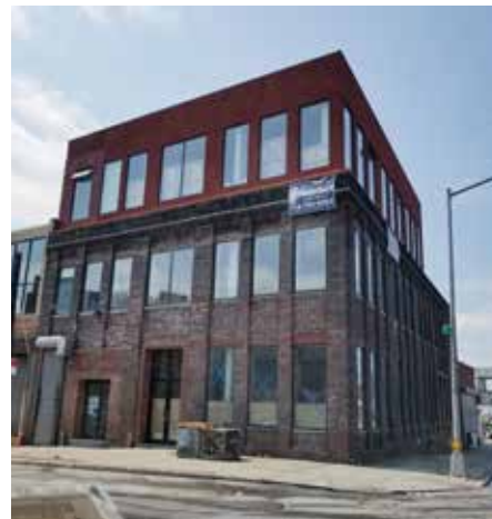
Enlarged building at the corner of 4th Street and Hoyt Street
