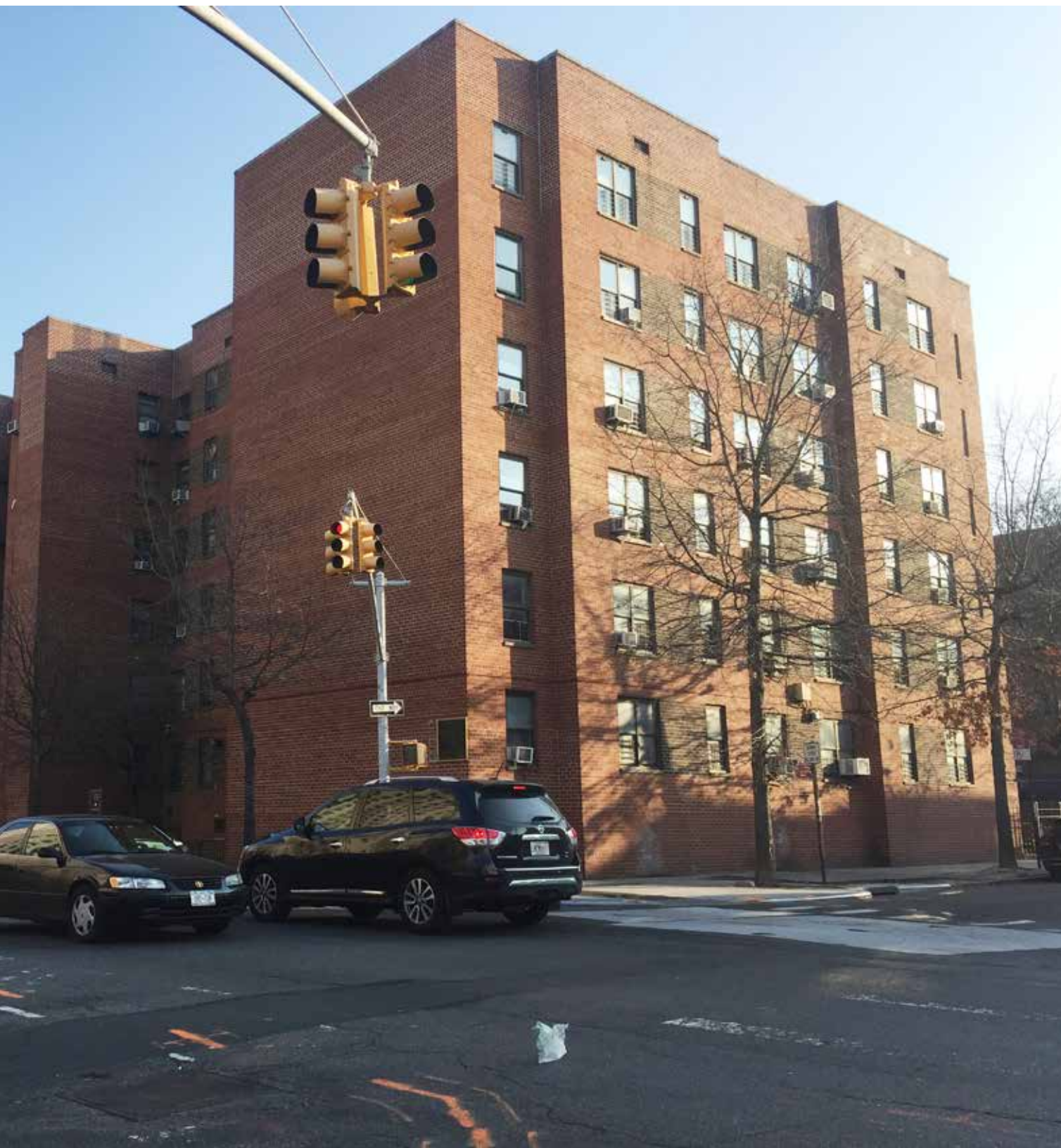
NYCHA Warren Street Houses
