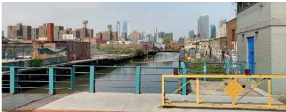
Looking north from Union Street bridge, Source: Cyclomedia
