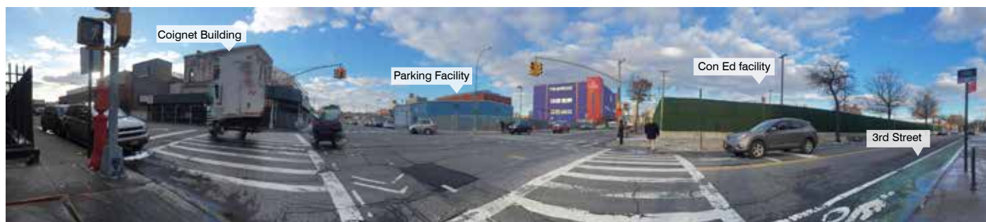
Intersection of 3rd Street and 3rd Avenue
