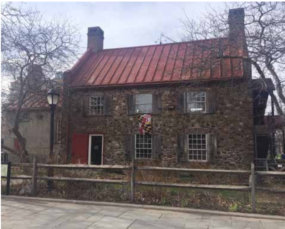
The Old Stone House in J.J. Byrne Playground
