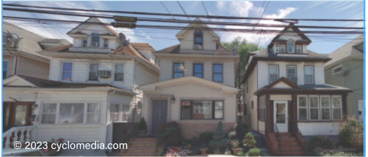
139-44 87th Avenue, Queens
