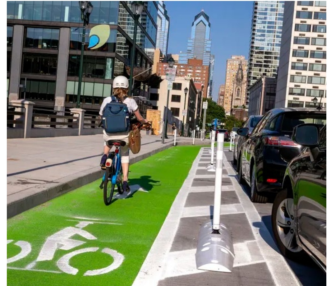
Protected Bike Lane on Bedford Avenue
