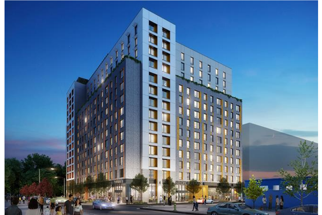
Chestnut Commons 274-units of 100% affordable housing in East New York opened in 2022
