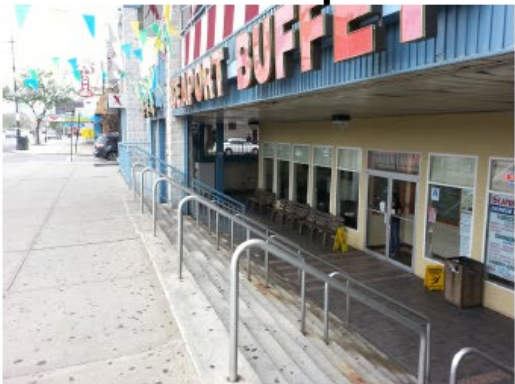
Below grade retail space in cellar
