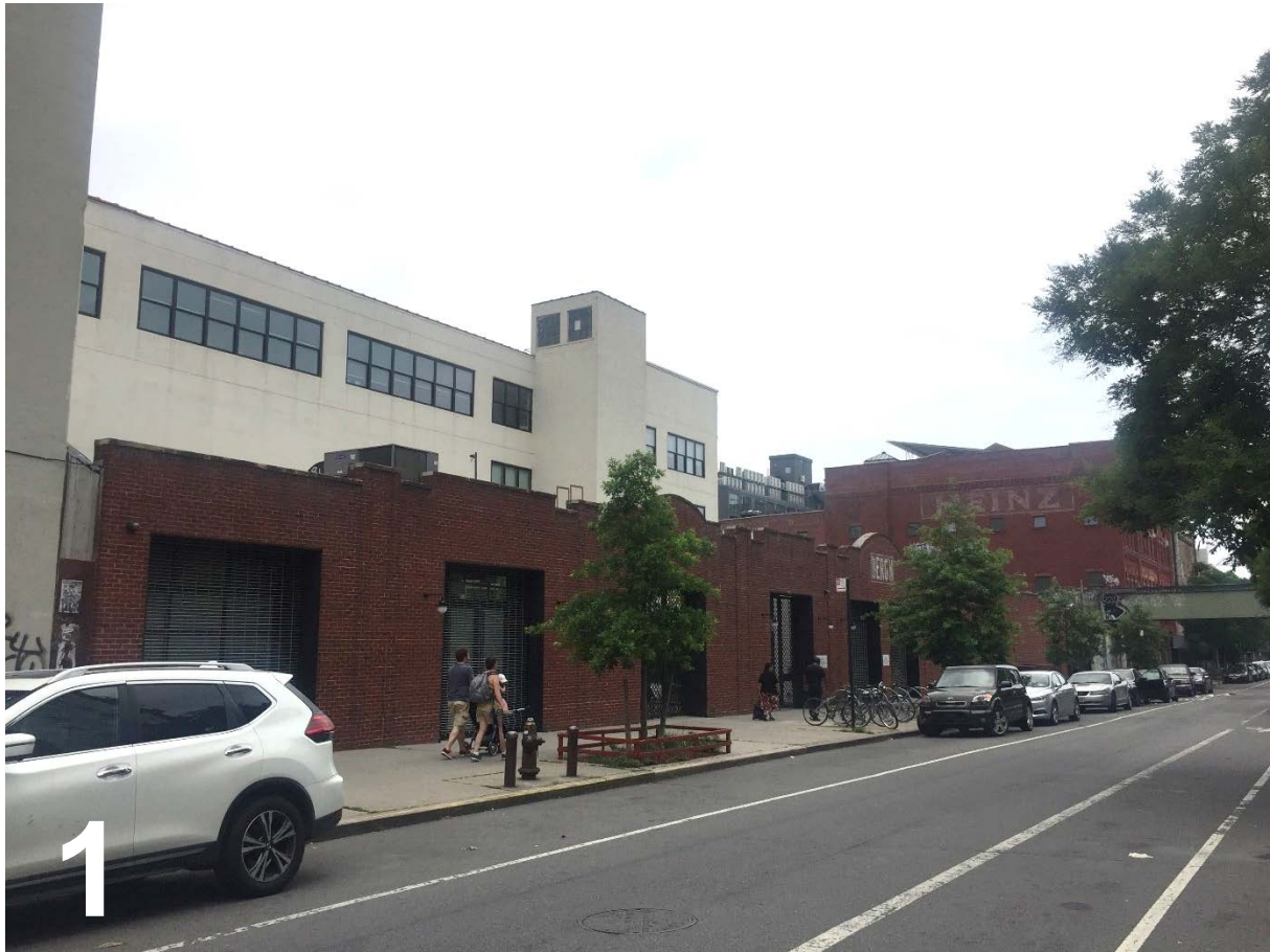
View of Bergen St (looking east towards Franklin Ave)
