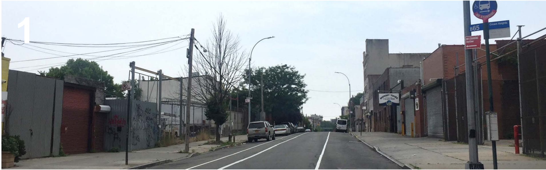
View of Dean St (looking east near Grand Ave)
