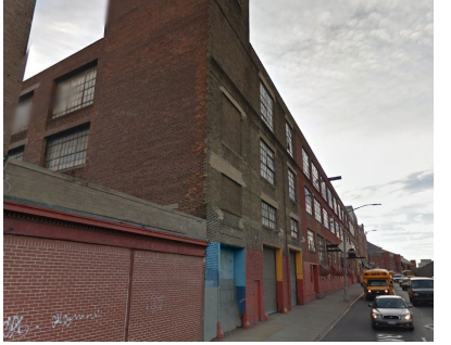
Studio E Warehouse
