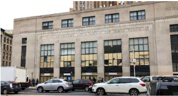
Long-vacant, two-story, 20,000 SF historic property.
