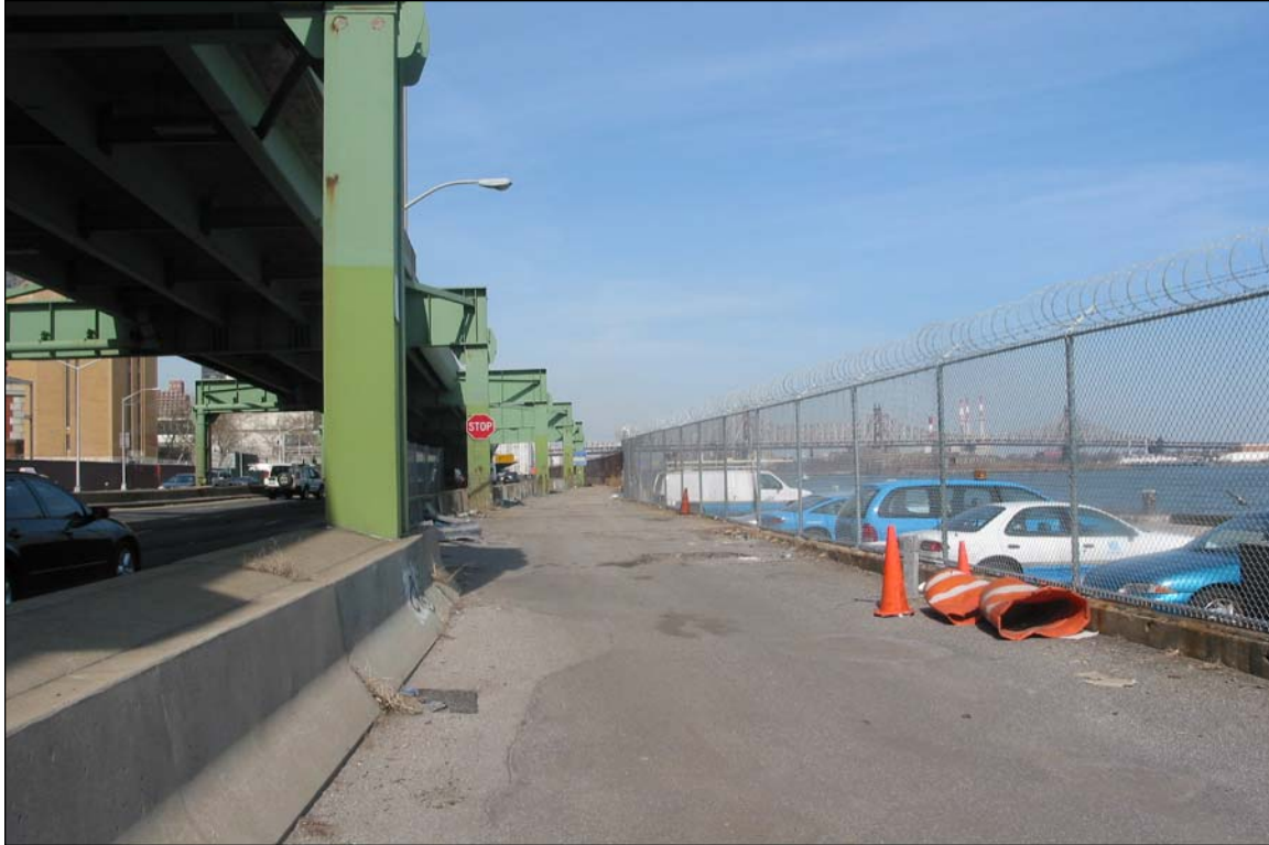
Photo 28: Roadway alongside parking pier ending at 41st Street
