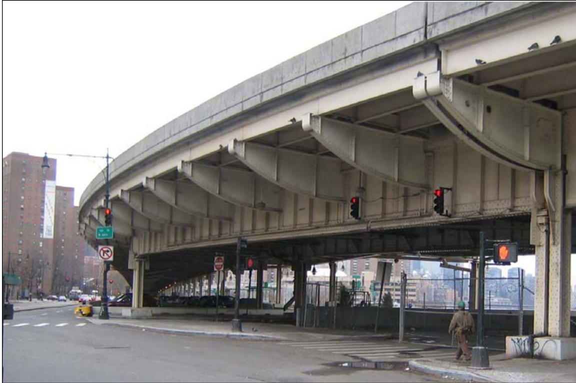
Photo 7: FDR Drive viaduct at Stuyvesant Cove Park
