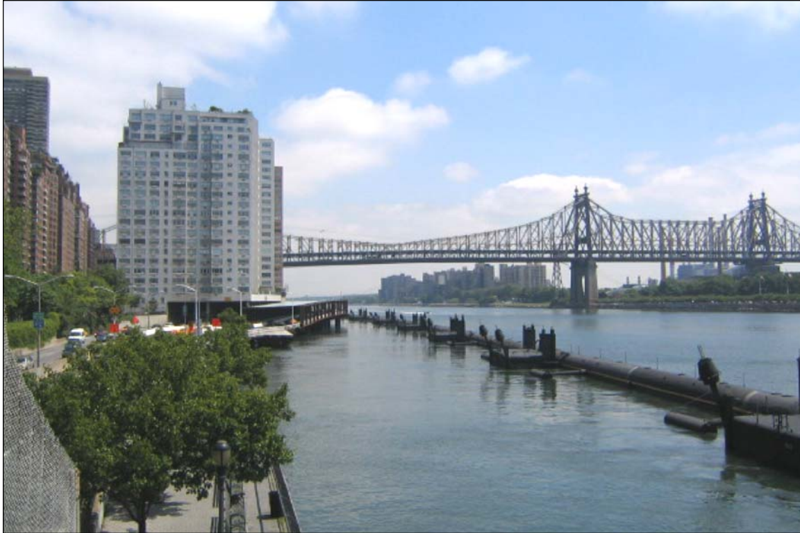
Photo 8: View of Queensboro Bridge looking north towards Sutton Place (ODR now dismantled)
