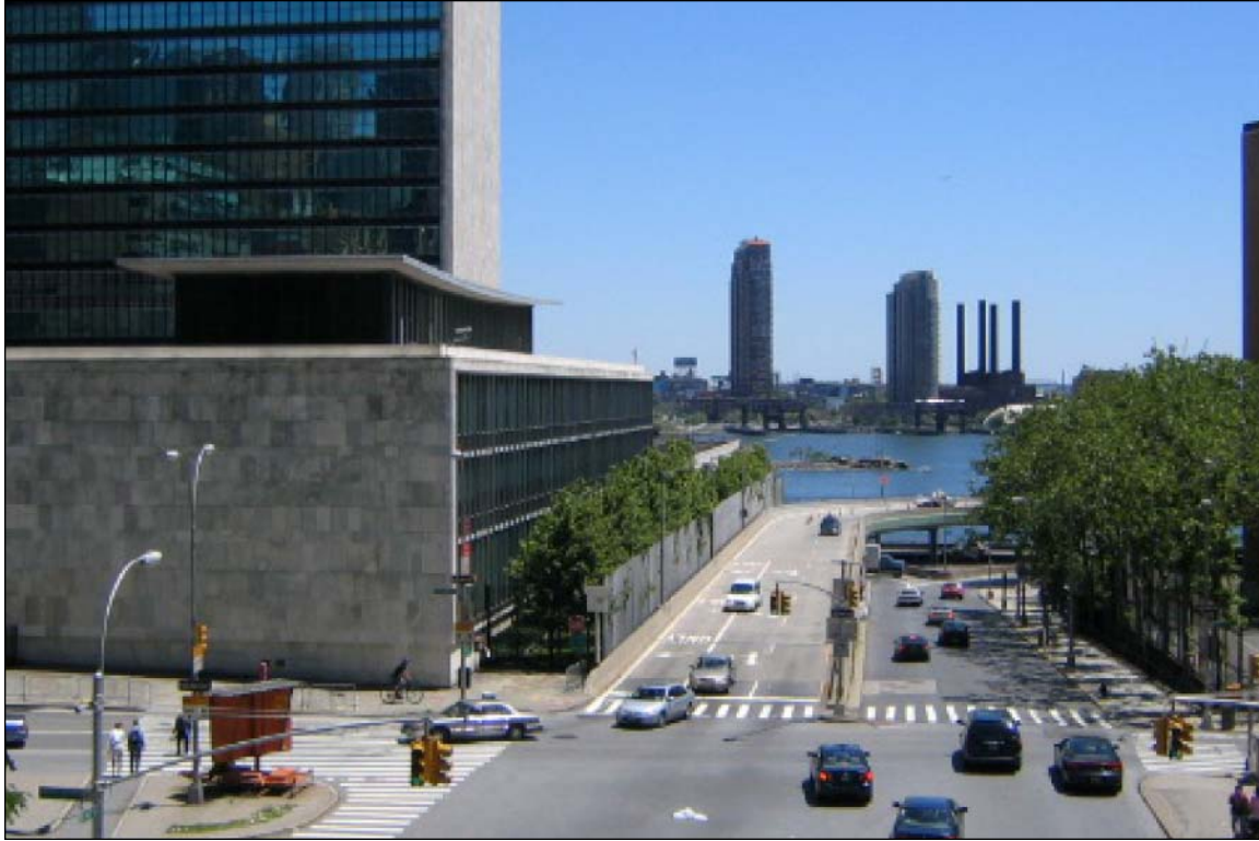
Photo 11: View east to the elevated FDR Drive 42nd Street off-ramp next to United Nations
