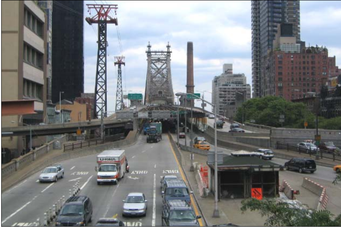
Photo 12: View of Queensboro Bridge looking east from 60th Street and Second Avenue
