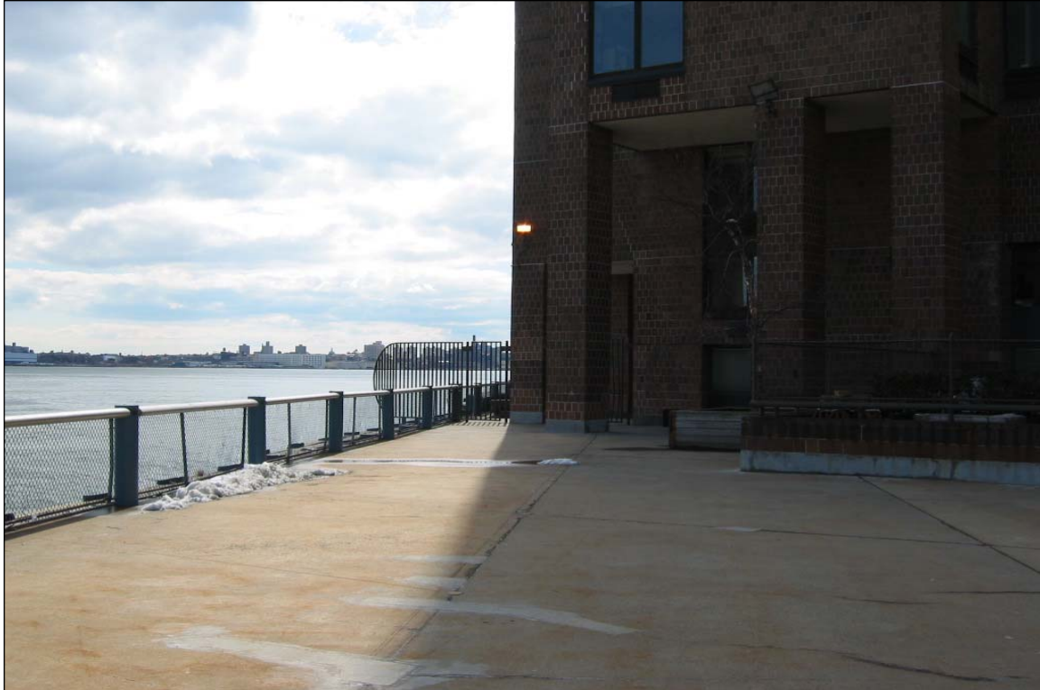
Photo 25: View south to closed walkway at Waterside Plaza
