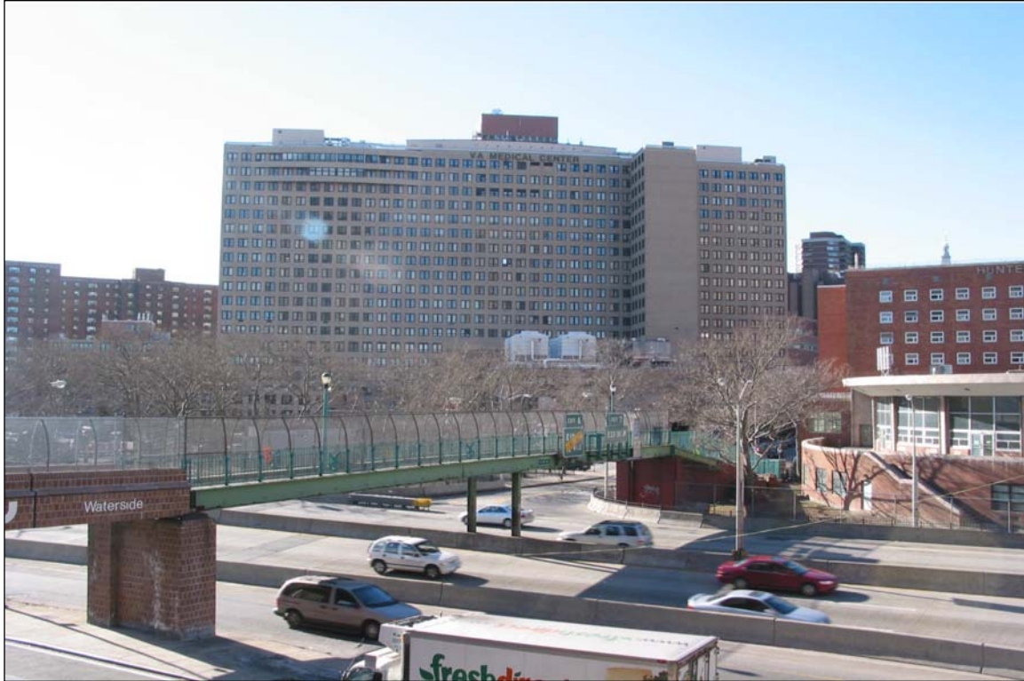
Photo 22: Pedestrian overpass bridge at East 25th Street, view from Waterside Plaza
