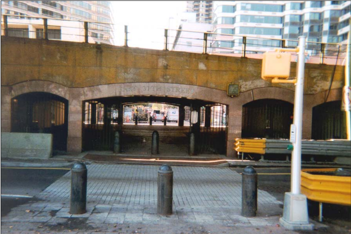
Photo 23: Pedestrian underpass from Glick Park at 37th Street
