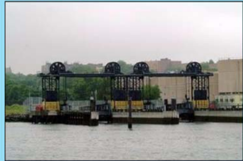
Rail float bridges - 65 th Street Rail Yard (Photo: Bernard Ente)
