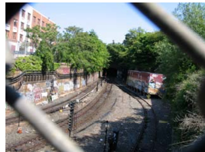
38 th Street rail cut
