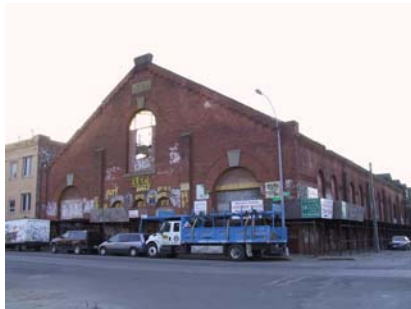
E. W. Bliss building
