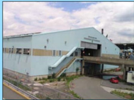
Hamilton Avenue Marine Transfer Station (Photo: DCP)
