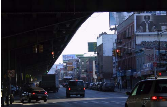
Third Avenue under the viaduct
