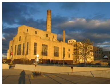
BAT boiler building – potential brownfield
