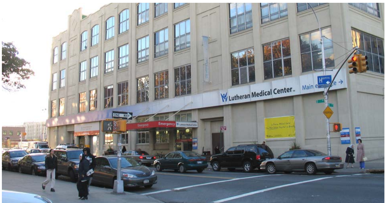
Lutheran Medical Center on Second Avenue and 55 th Street
