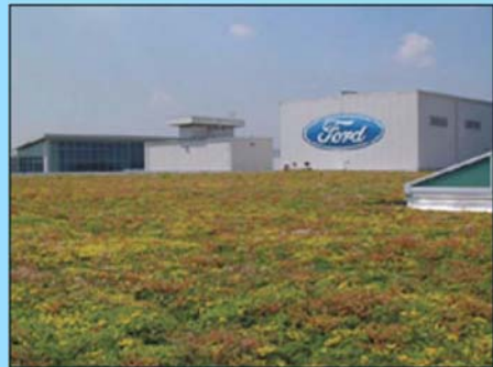
Green roof - Ford Dearborn Truck Assembly Plant, Michigan, W. McDonough + Partners, Architects
