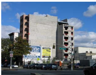
Fourth Avenue and 21 st Street
