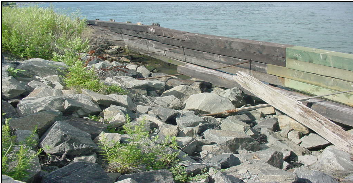
Figure 16-4: Existing Bulkhead Along Western Edge of Project Site
