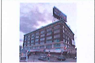
6. The Paragon Oil Building
