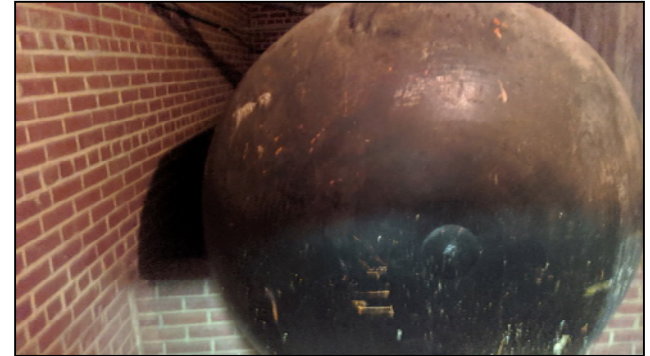
Photograph 2. 2,000-gallon diesel AST located in the basement.
