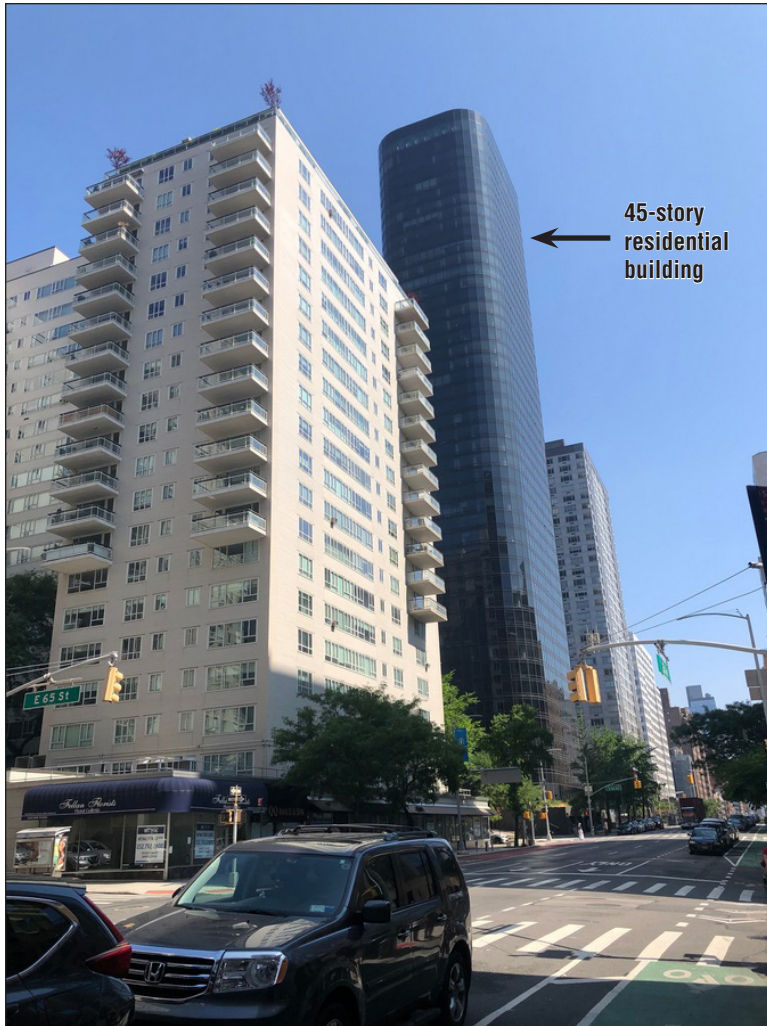
View north on Second Avenue, showing the Manhattan House, 265 East 65th Street, and 1283 Second Avenue
