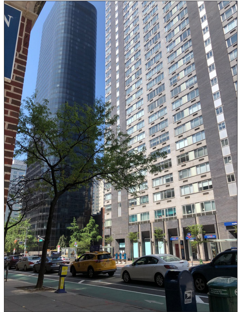
View southwest on Second Avenue to the 45-story residential building at 265 East 65th Street in the Rezoning Area, with the apartment tower at 1283 Second Avenue to the right; both buildings face Second Avenue 4
