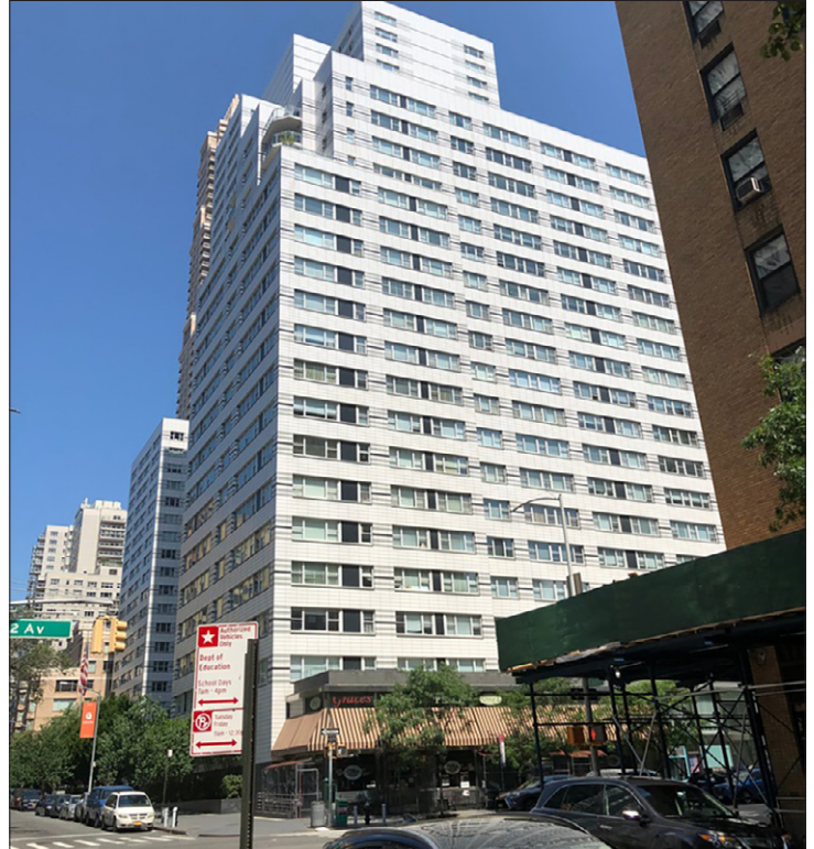
View northwest to the apartment building at 215 East 68th Street/ 1299 Second Avenue 8
