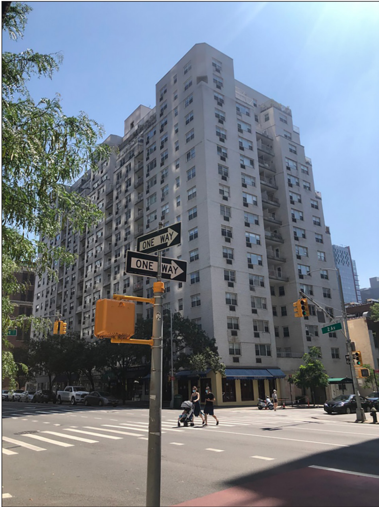
View northeast on Second Avenue to the Rezoning Area building at 301 East 66th Street 3
