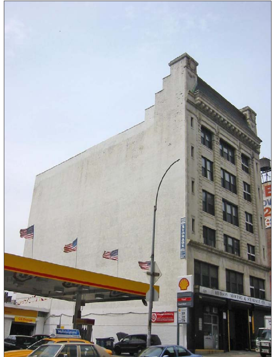
Sheffield Farms Stable – south facade
