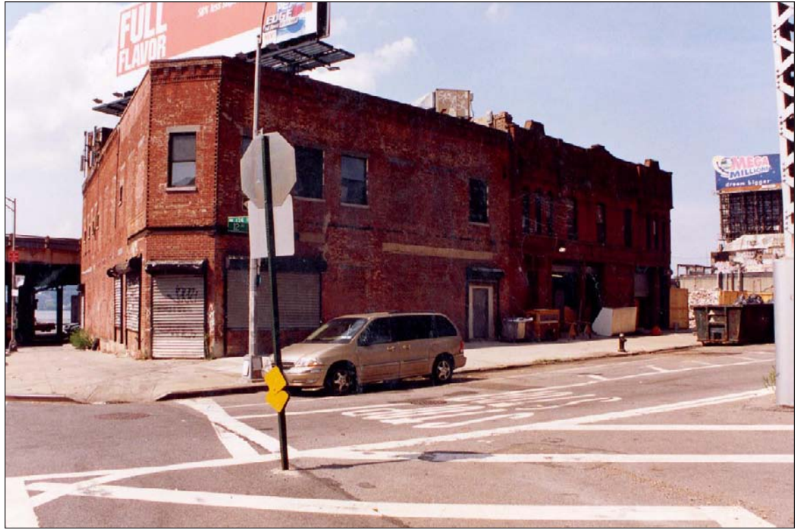
Block 2004. View west at Twelfth Avenue and 125th Street 35
