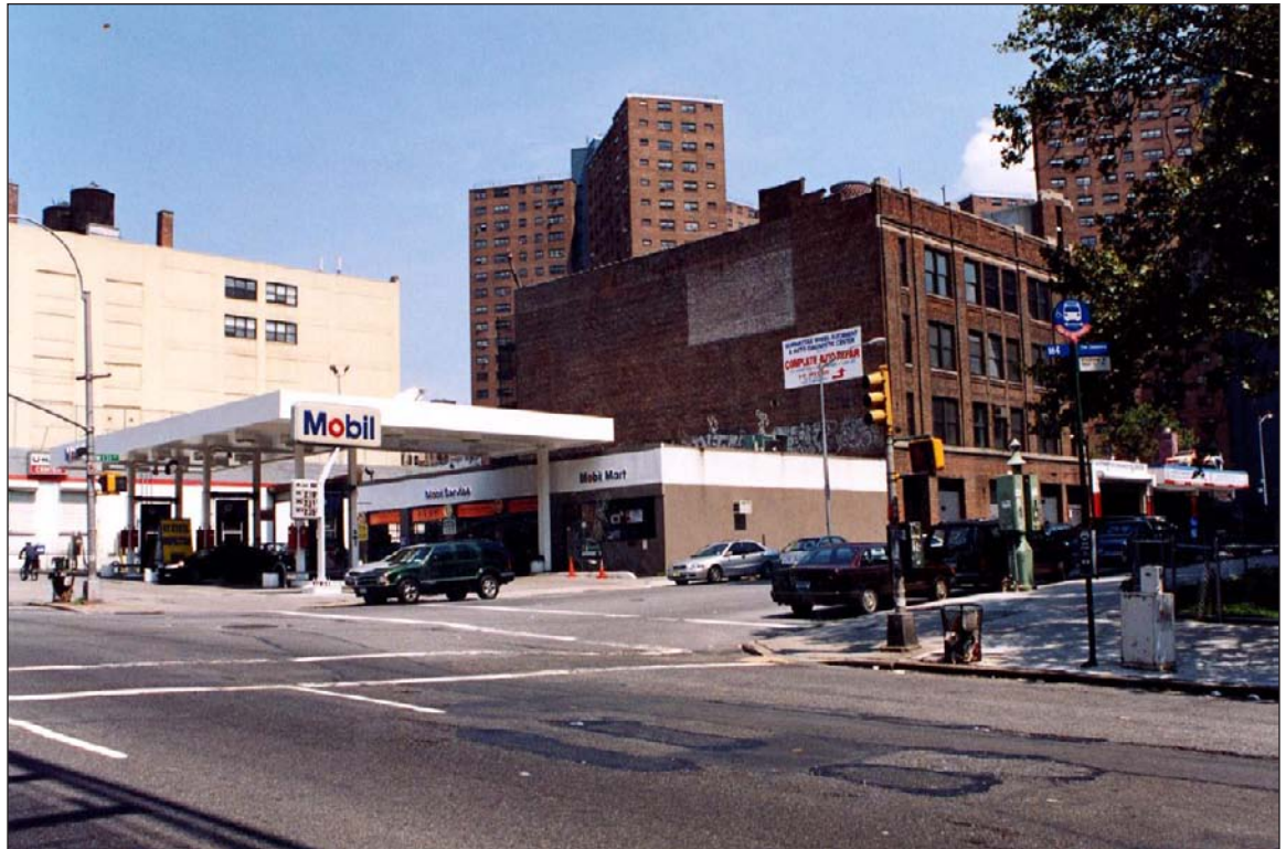
Block 1986. View northeast from Broadway and 131st Street 24
