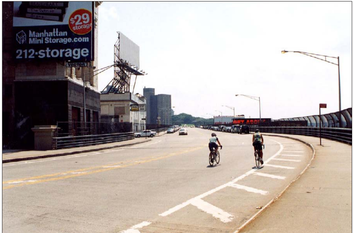
Riverside Drive viaduct. View south from 135th Street 30
