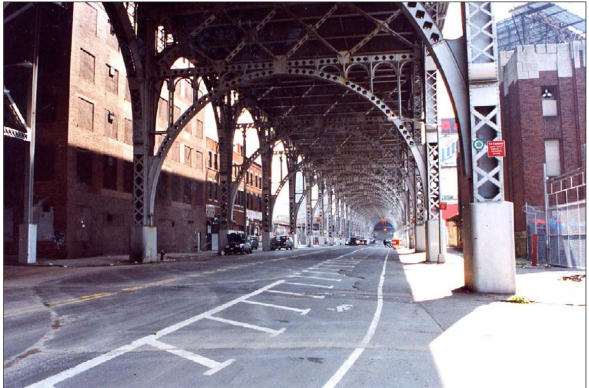
Riverside Drive viaduct. View south on Twelfth Avenue from 134th Street 4
