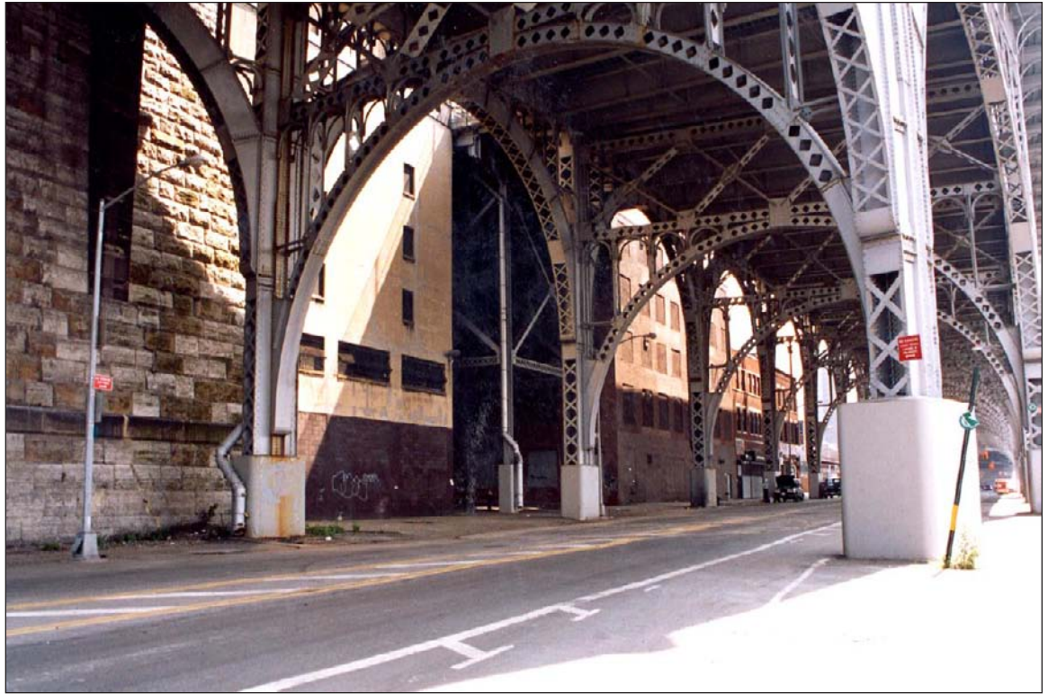
View southeast on Twelfth Avenue from the vicinity of 134th Street 37
