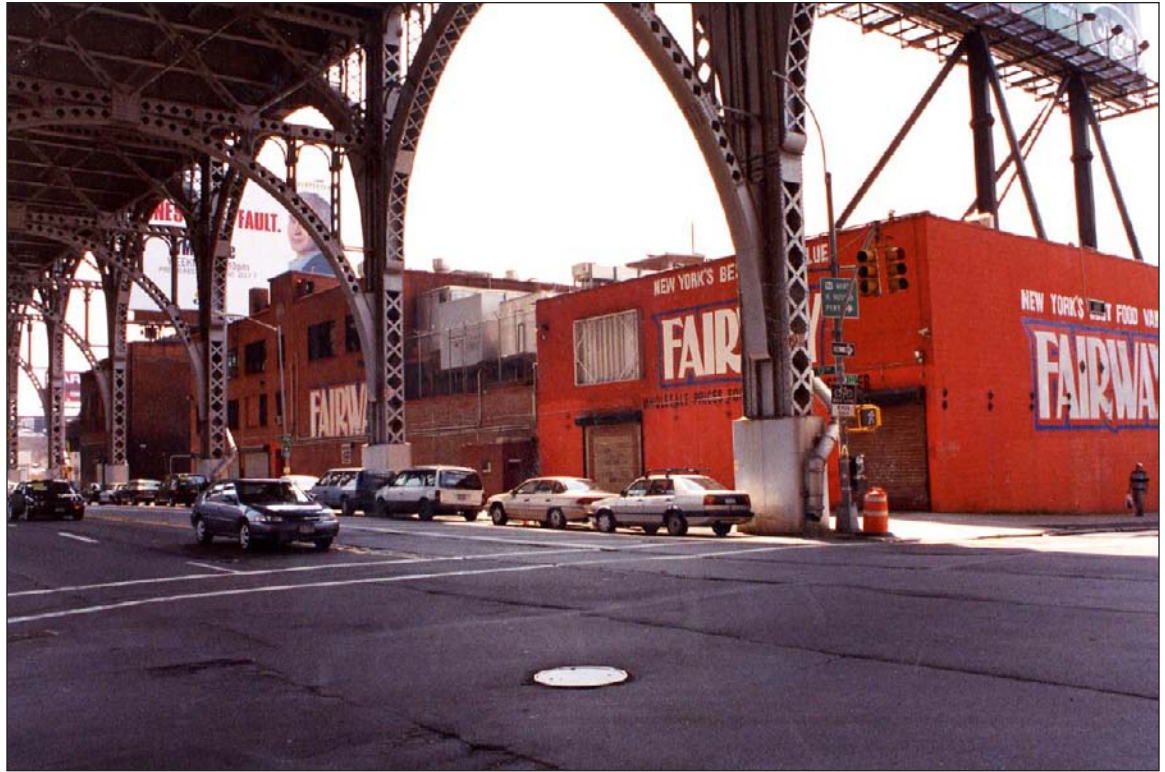
Block 2004. View southwest on Twelfth Avenue from 133rd Street 33
