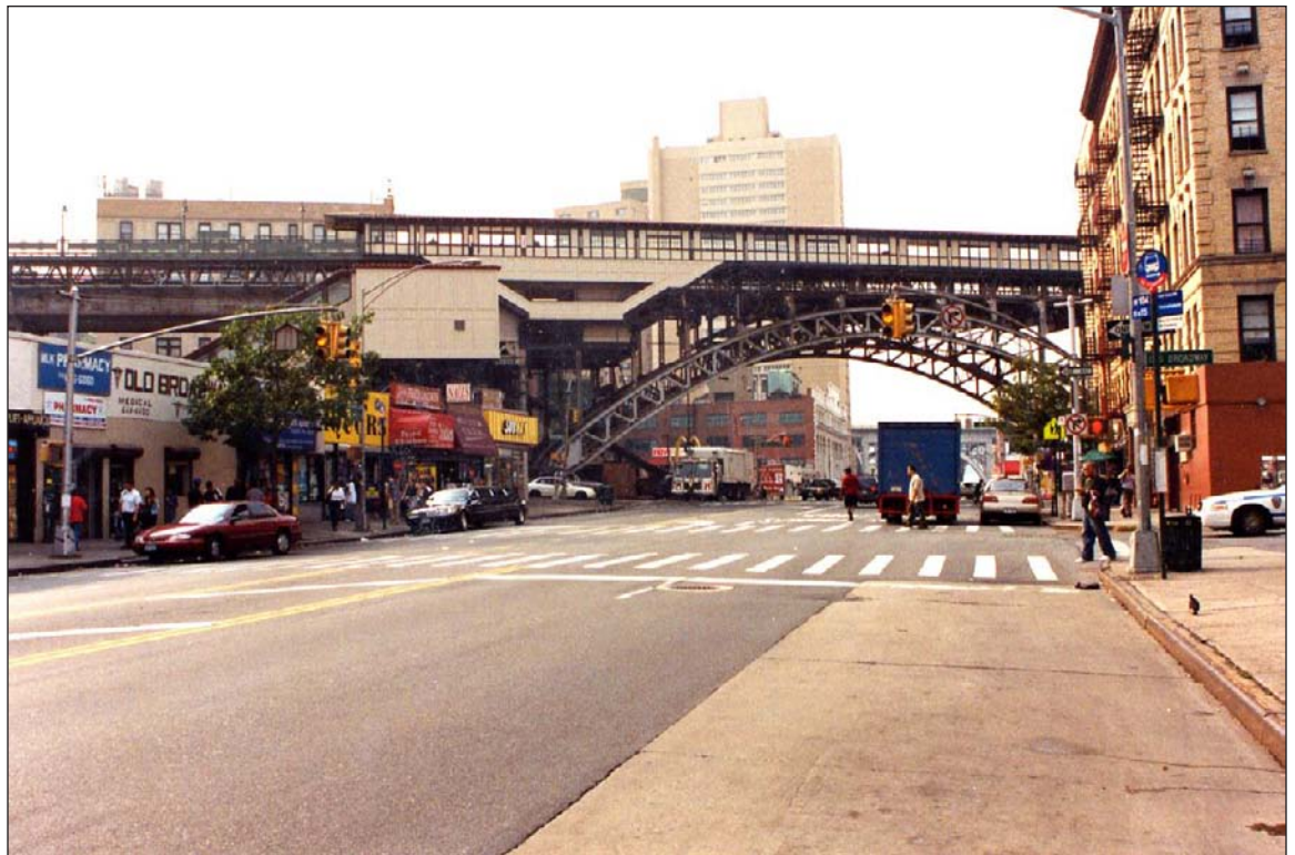
Manhattan Valley IRT viaduct. View west on 125th Street 2
