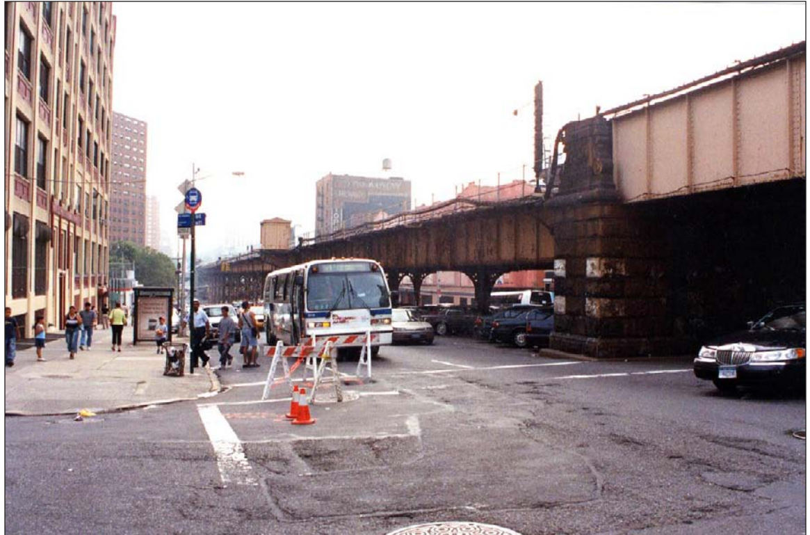
Manhattan Valley IRT viaduct. View south on Broadway from 133rd Street 3
