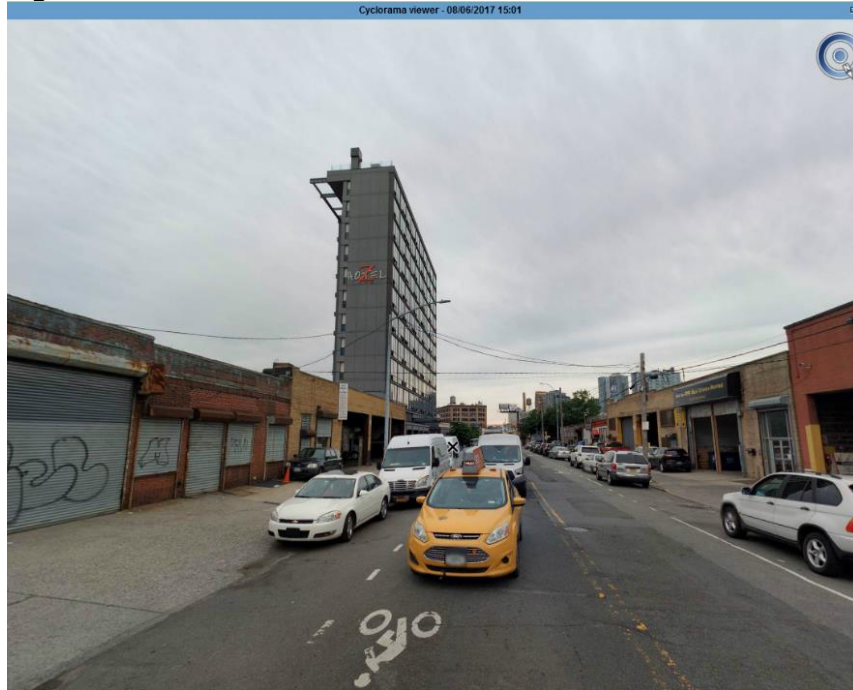
Figure 1-6 Hotel in Active Industrial Area (LIC)
