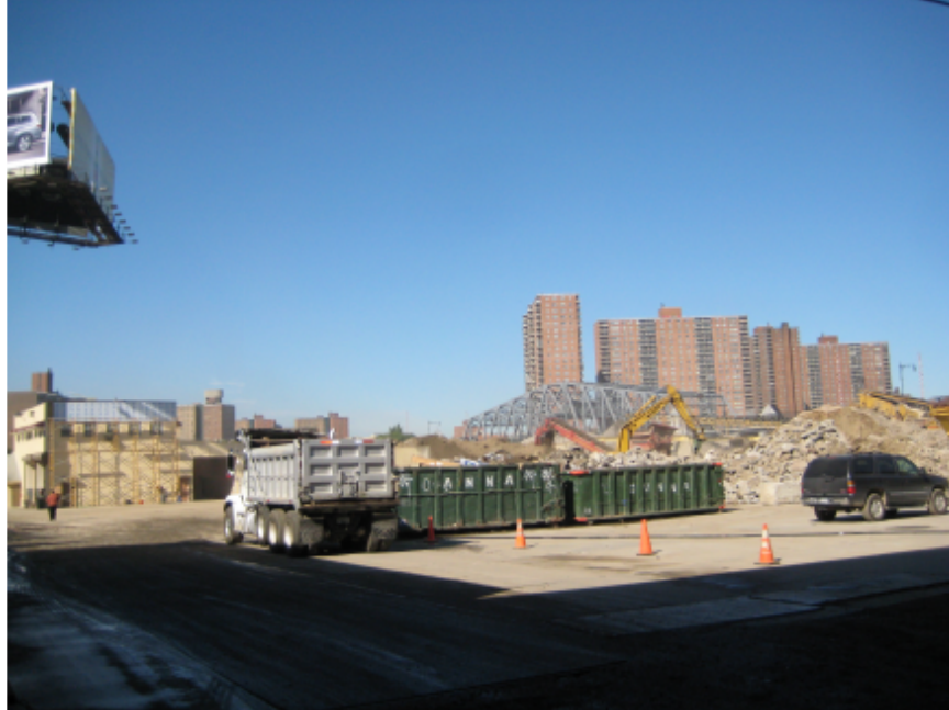
RWCDs Site #1 viewed looking west from Exterior Street.
