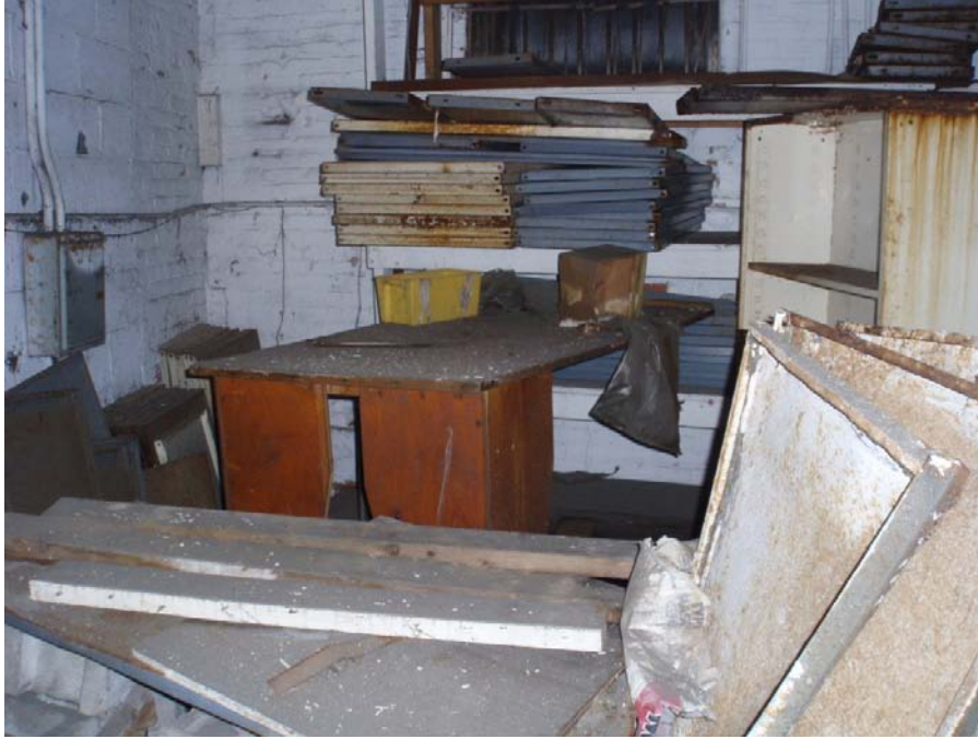
Photograph 9 – Miscellaneous Trash - Building No. 1
