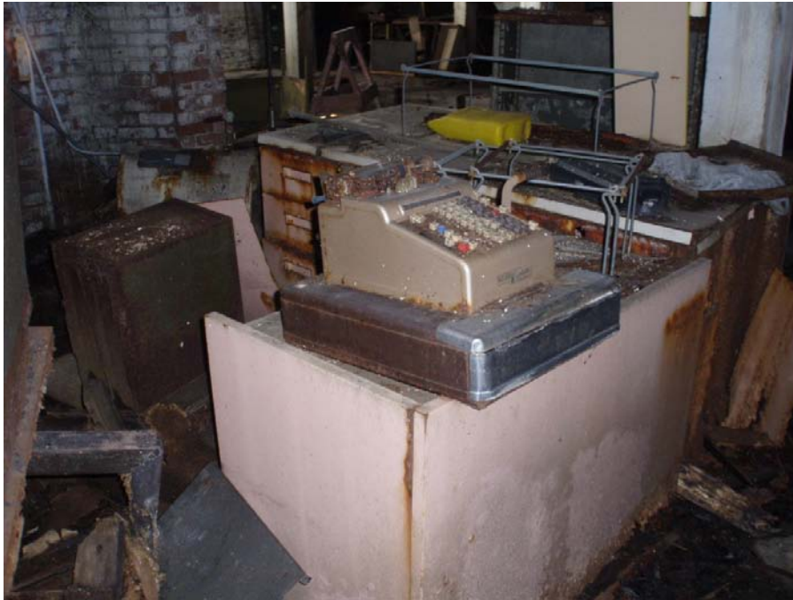
Photograph 10 – Miscellaneous Trash - Building No. 1
