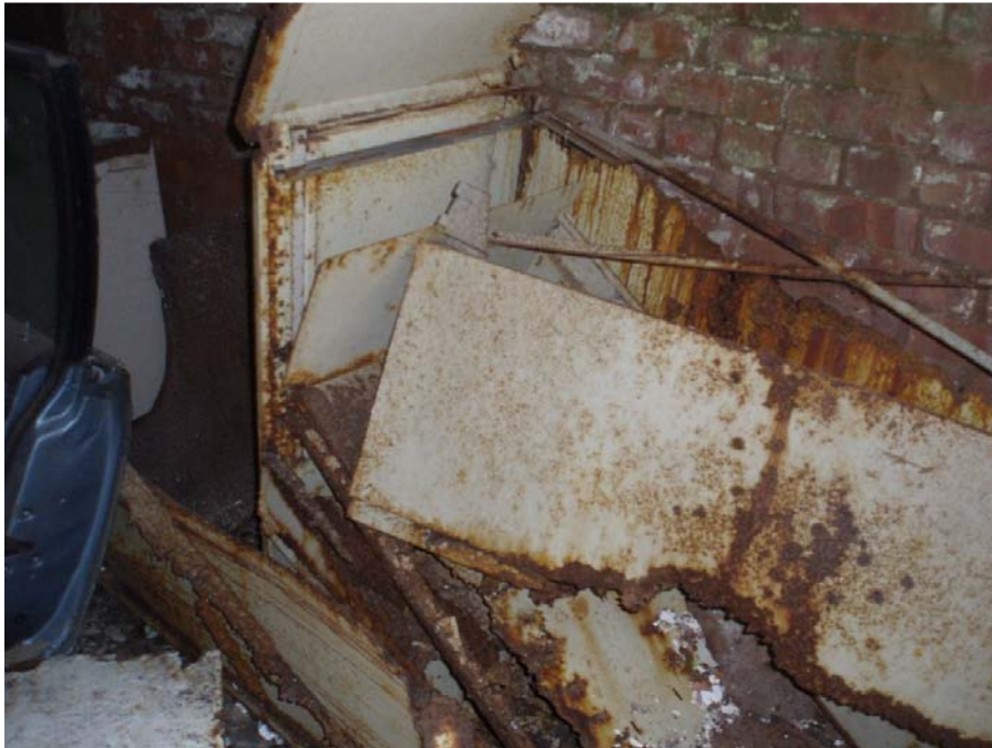
Photograph 20 – Miscellaneous Trash – Building No. 1
