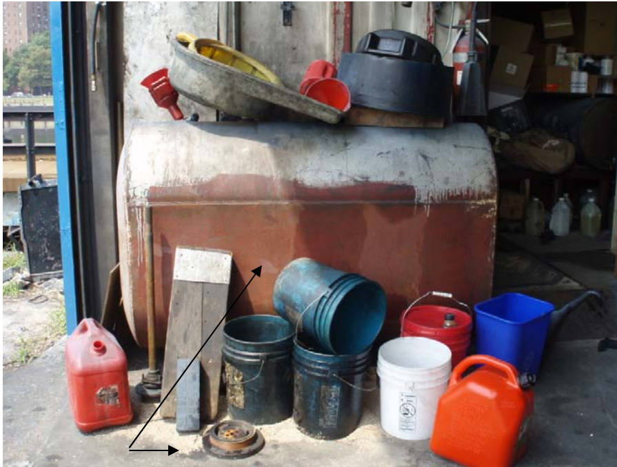
Photograph 38 – Above Ground Storage Tank and Spill – Garage
