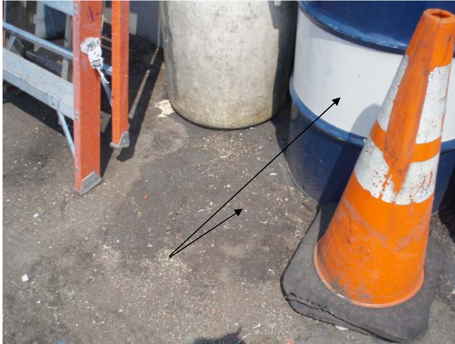
Photograph 61 – Drum and Stain Beneath Drum Near Garage on Lot 28
