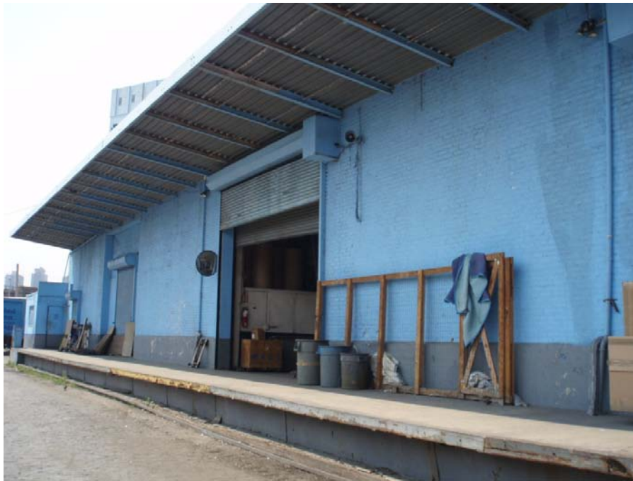
Photograph 26 – Access to Building No. 2
