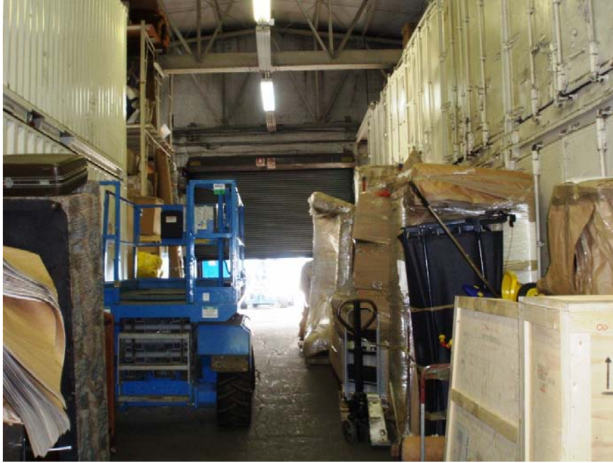
Photograph 37 – Fluorescent Lights – Building No. 2
