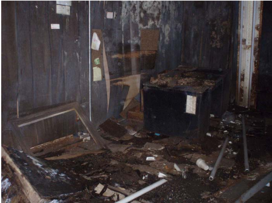
Photograph 8 – Miscellaneous Trash - Building No. 1
