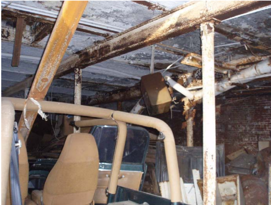
Photograph 24 – Miscellaneous Trash – Building No. 1
