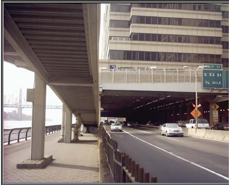
Figure 12-3. View looking south from under the public pedestrian ramp.
