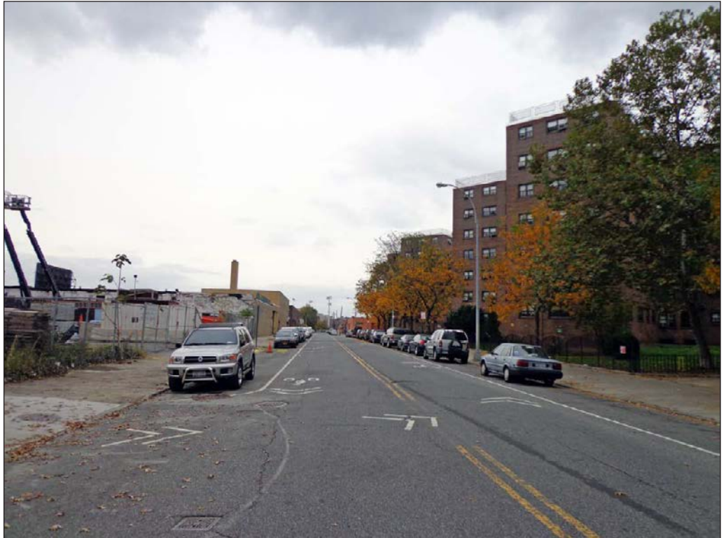
North view along 1st Street from Astoria Boulevard of the parking area and structure located on Block 490 of the WF Parcel 3
