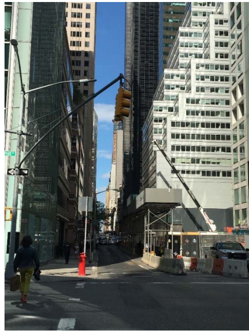
Photo 6: View of the built context along East 56th Street, looking west from Park Avenue
